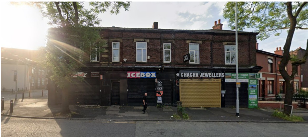
Picture B above showing the West Elevation fronting onto Heywood Street
