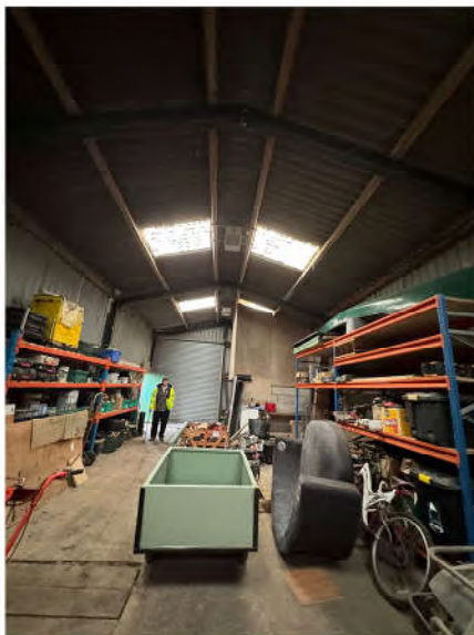
Inside adjacent barn to southwest
