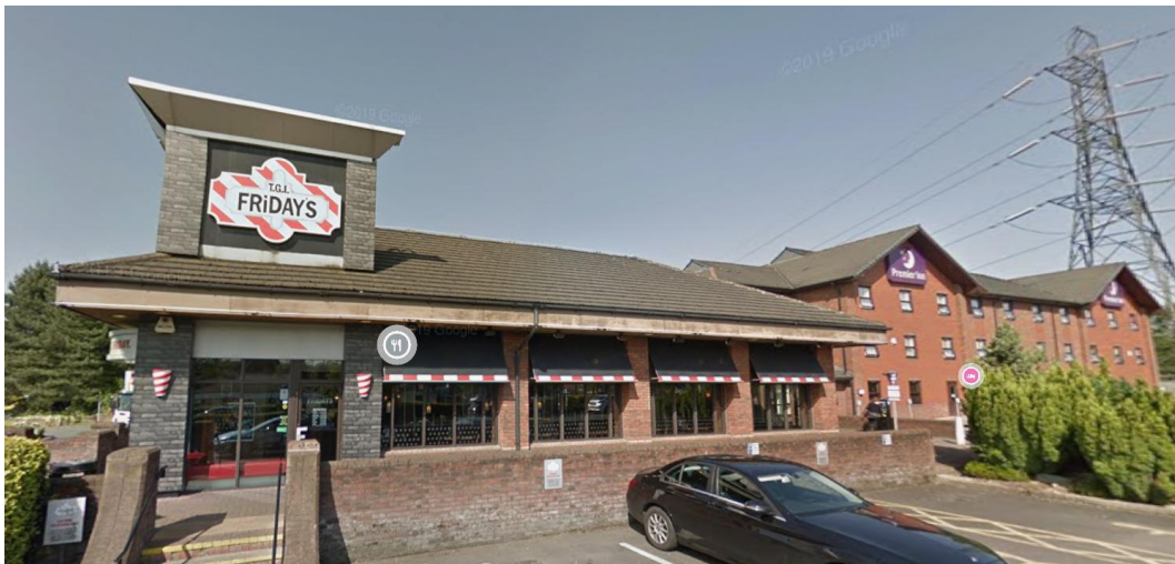
Figure 2. Side Elevation (Google Streetview)
