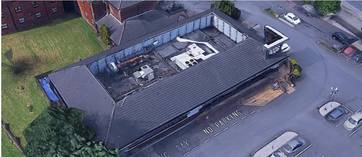
Figure 3. Satellite Image of Site's Mechanical Plant Area (Google Earth)
