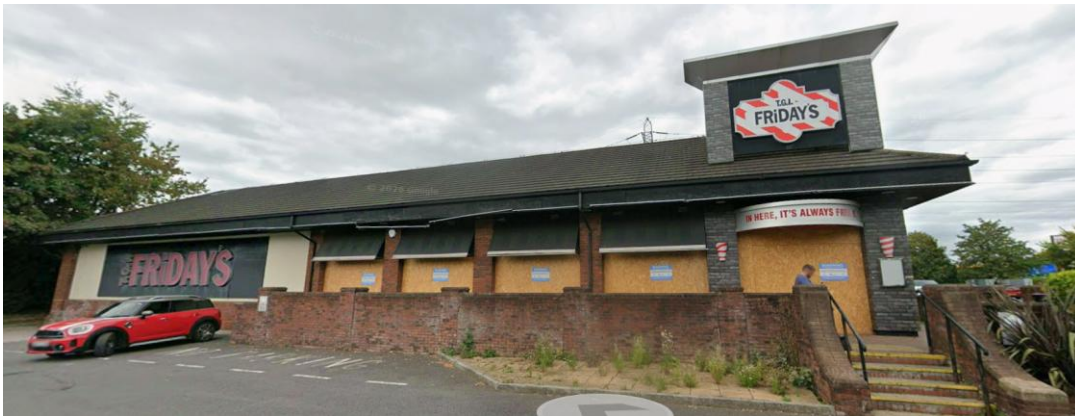
Figure 1. Application Site Frontage (Google Streetview)
