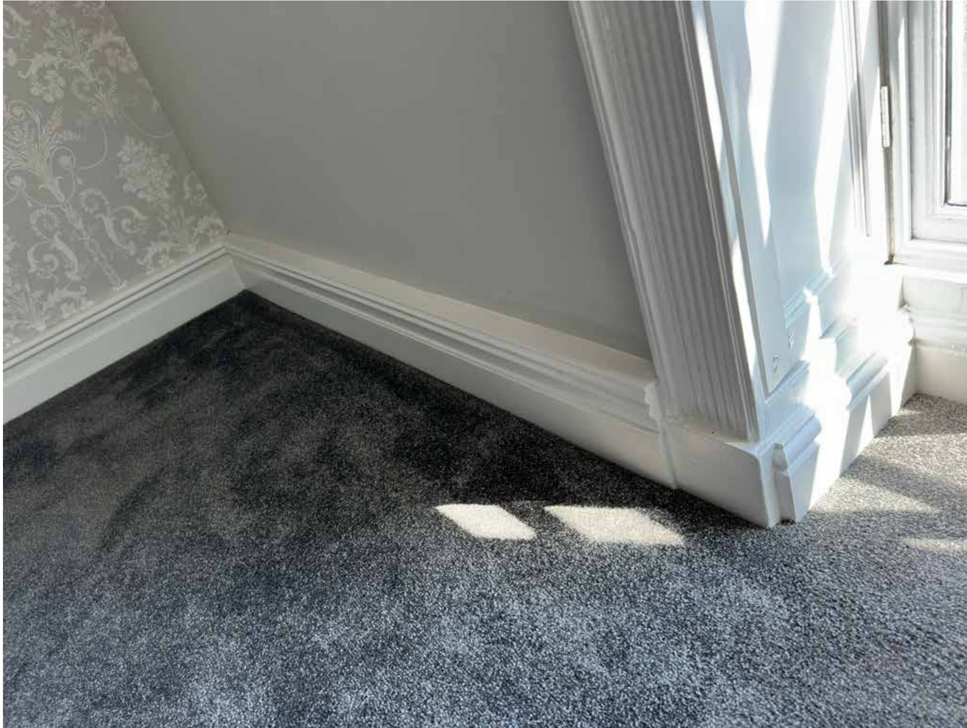
Figure 4: Photo of the skirting and architrave.
