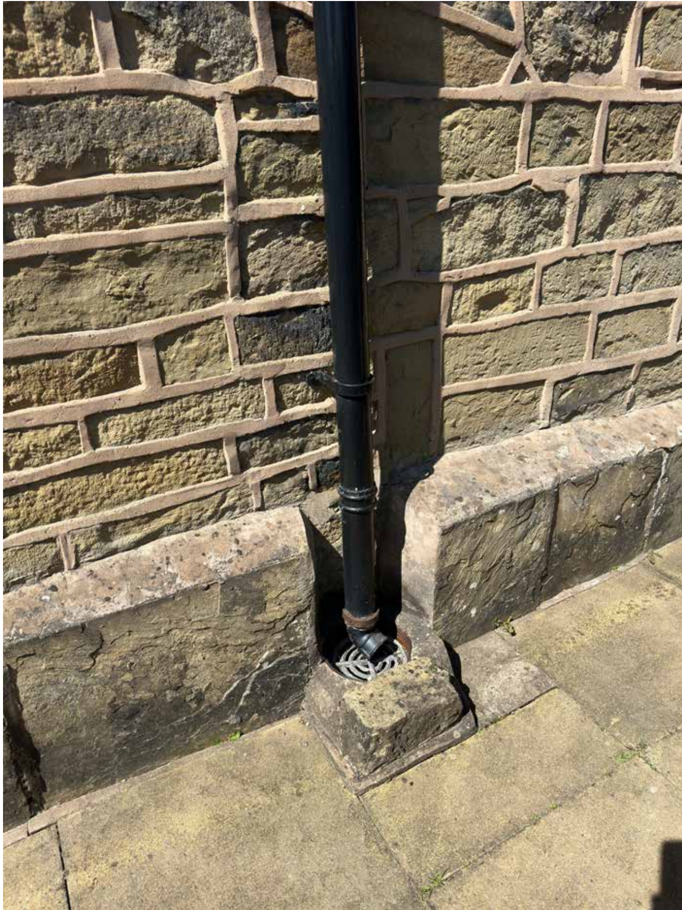
Figure 7: Existing cast iron rainwaterpipe on side elevation.
