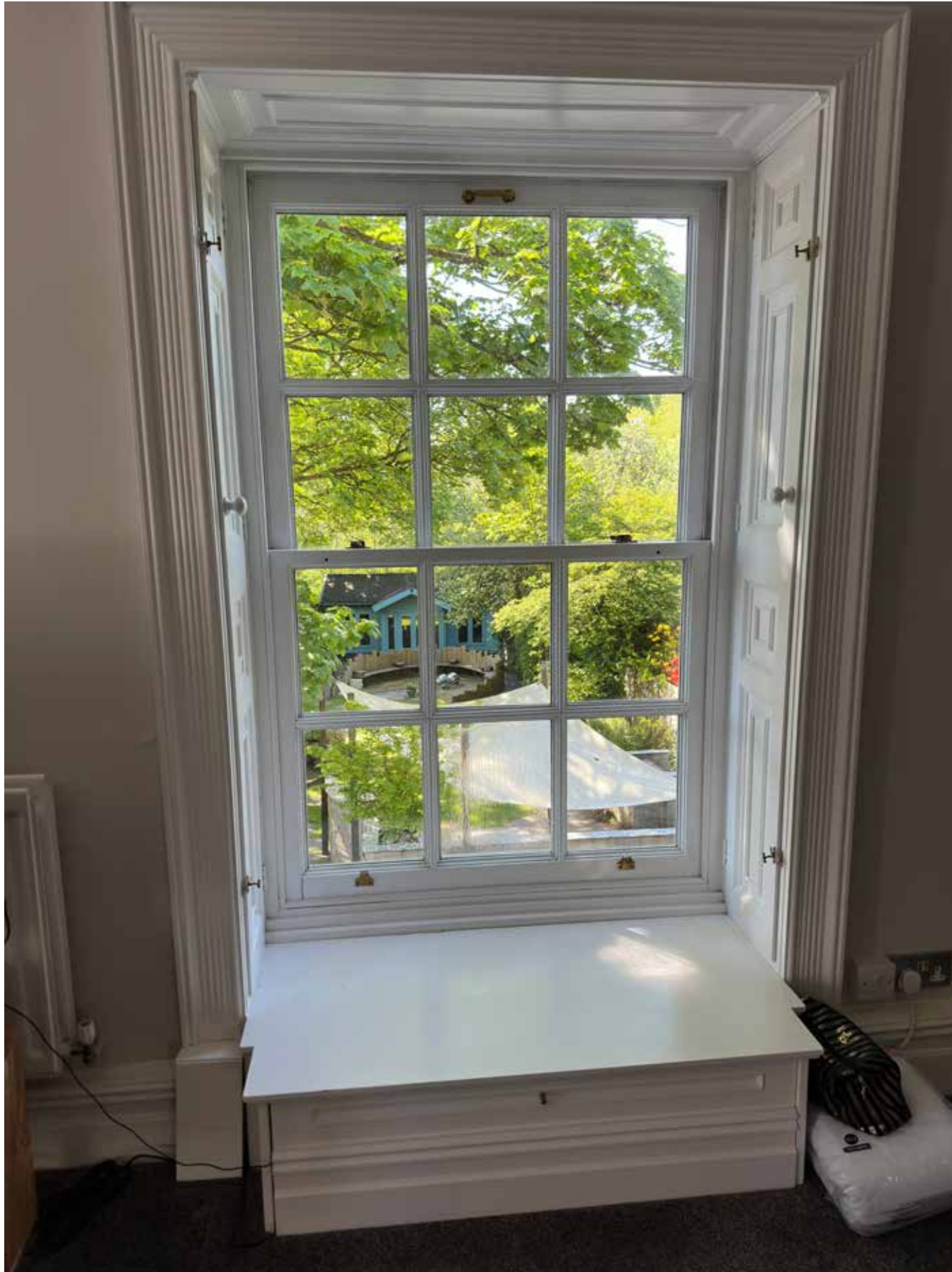
Figure 5: Sash Window on the front elevation with original features.
