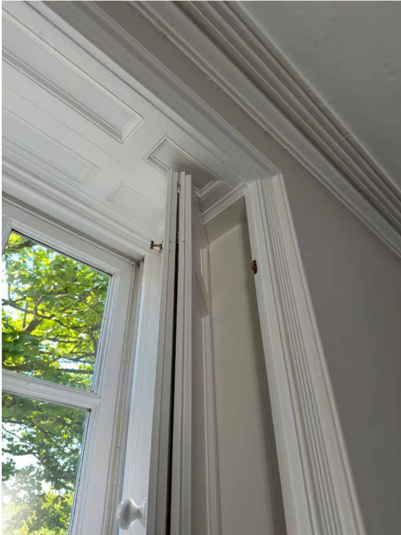
Figure 6: Closer view of original shutters & Architraving
