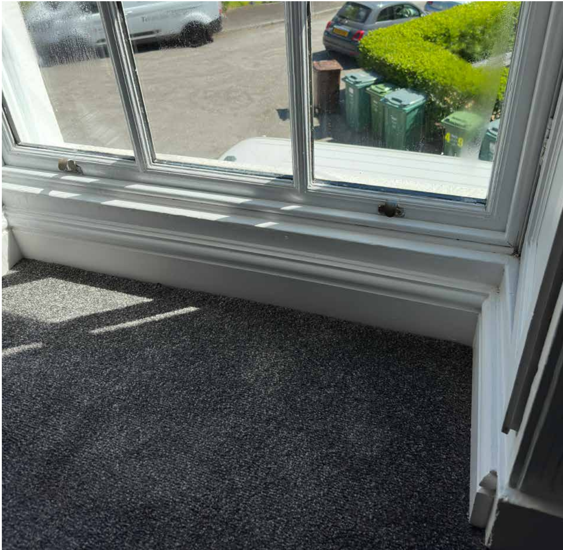
Figure 3: Closer view of the window.
