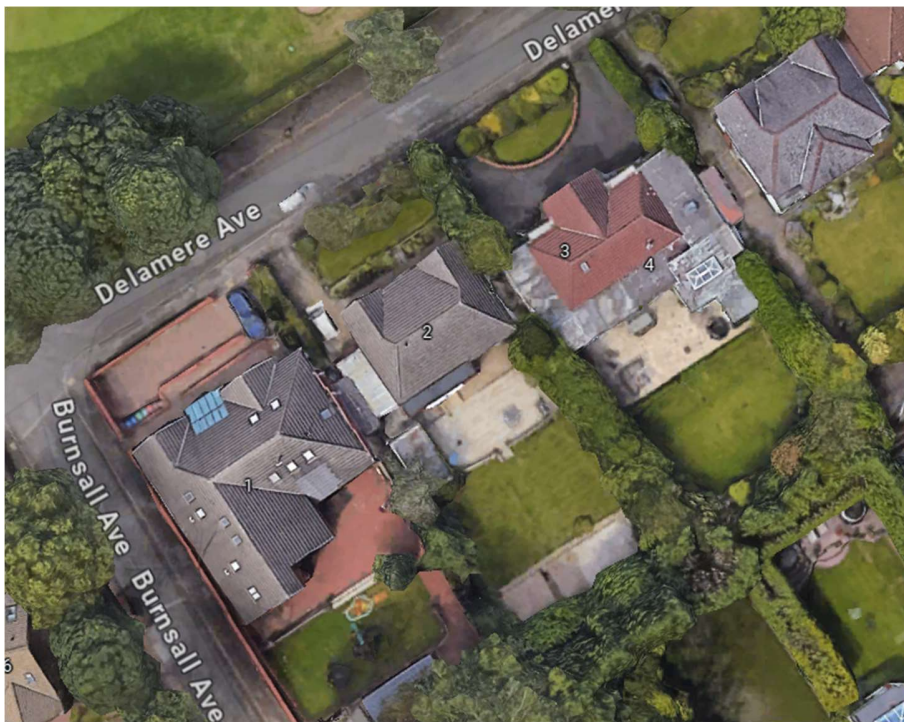
existing aerial view
