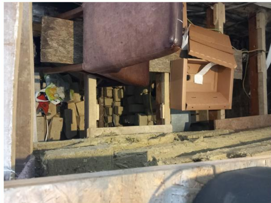
Photo No.6: Looking directly down from the ground-floor level to the underlying basement in the SW extent of the dwelling
