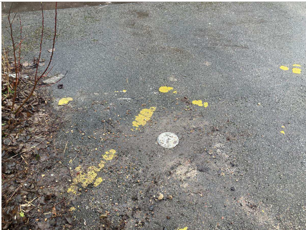
PLATE 6 WINDOW SAMPLE INSTALL CARPARK (WS103)
