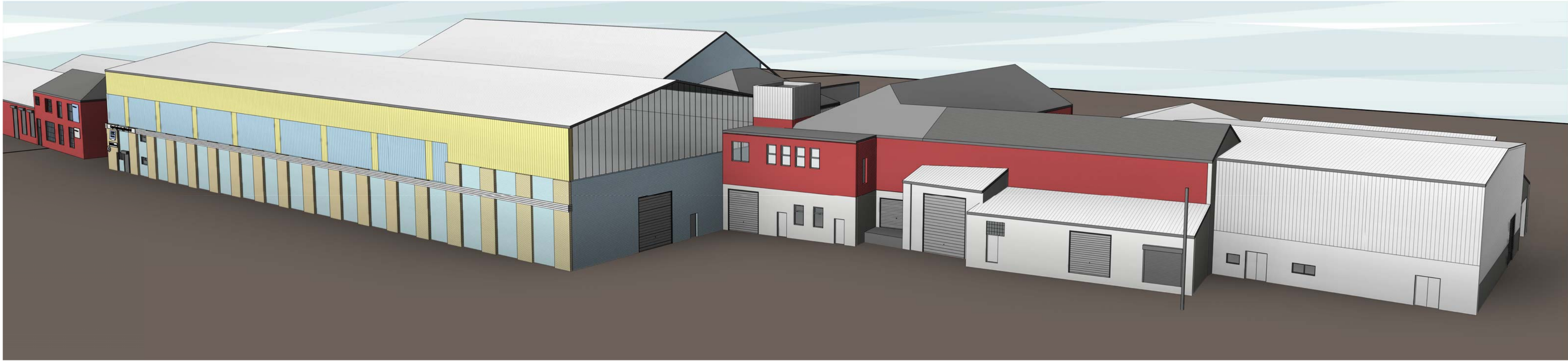
3. 3D - Existing View 3
