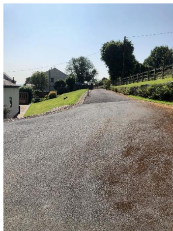
18. Road within Ferns Farm Site, looking towards the exit gate
