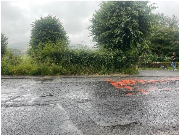
3. Access Rd from across Turton Rd Showing hedge
