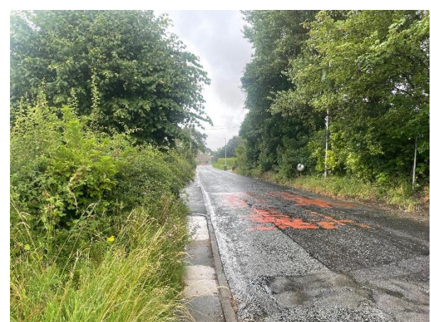
4. Access Rd from Turton Rd towards Tottington opp mirror
