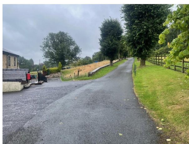
12. Access Rd from Site gate, 70m from Turton Rd
