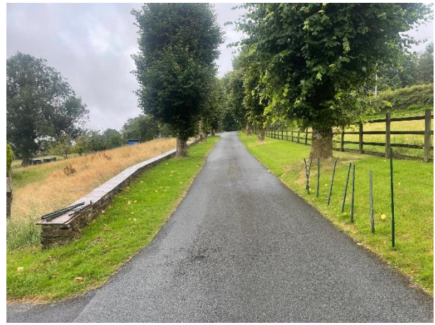
14. Access Rd 15 m from Site gate
