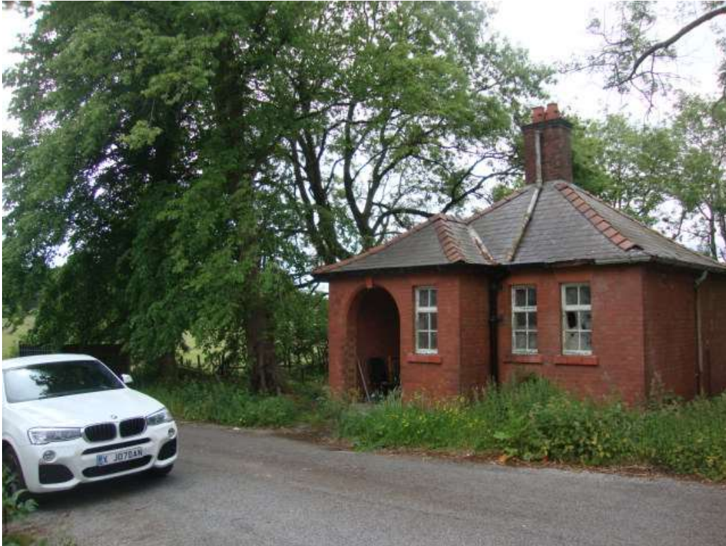
Plate 9 – Existing Gate House and southerly boundary to subject land
