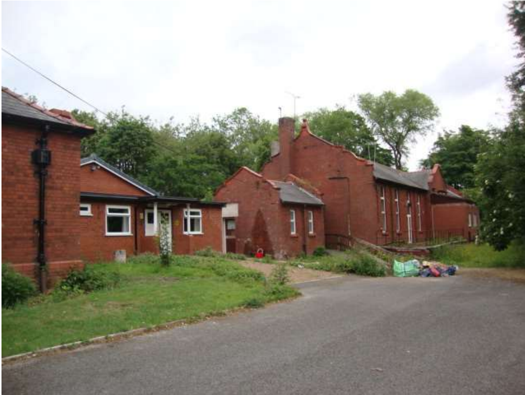
Plate 5 - View of Pavilion Block extending to east of site
