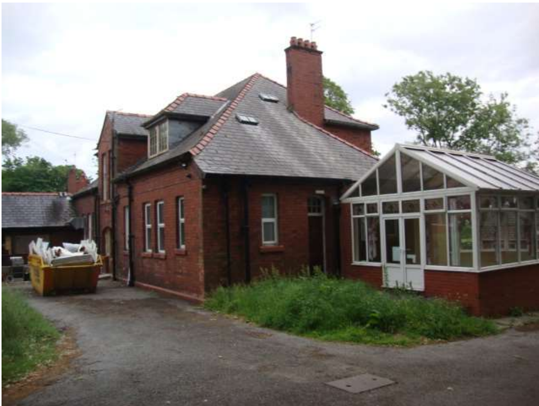
Plate 2 – Rear elevation of Administration Block
