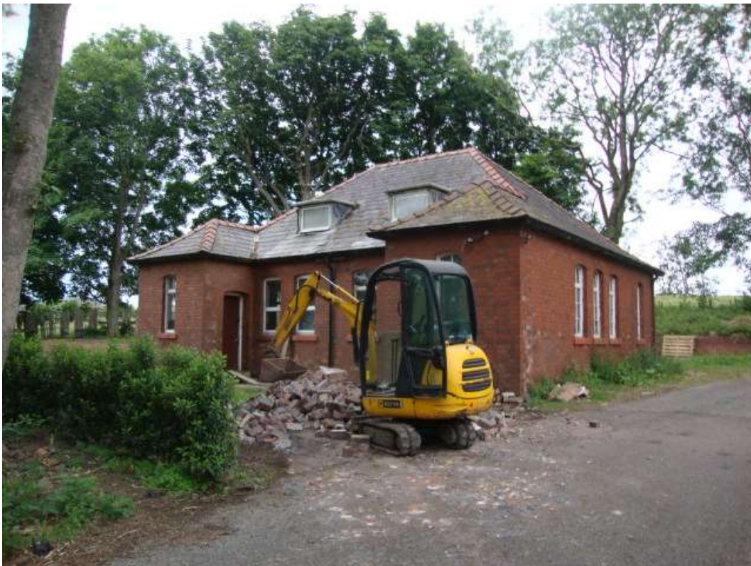
Plate 12 – View of the Wash House adjacent to north boundary of subject site.
