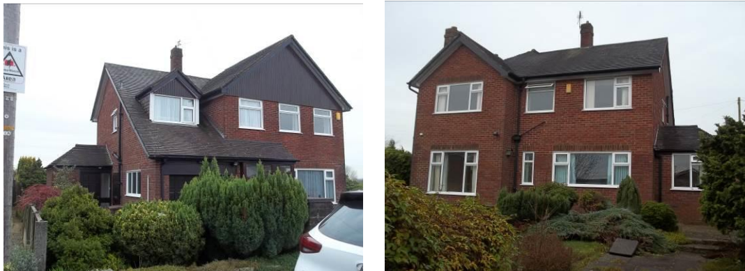
Front (west) and rear elevations
