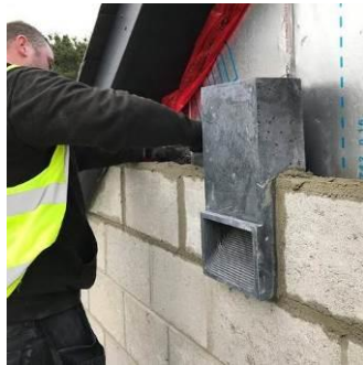
Green and Blue Bat Block/Brick in situ
