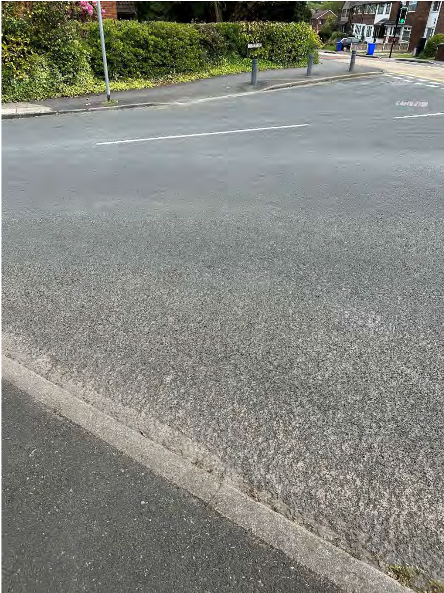
Photo 4 – Dropped Kerbs across Ainwick Drive
