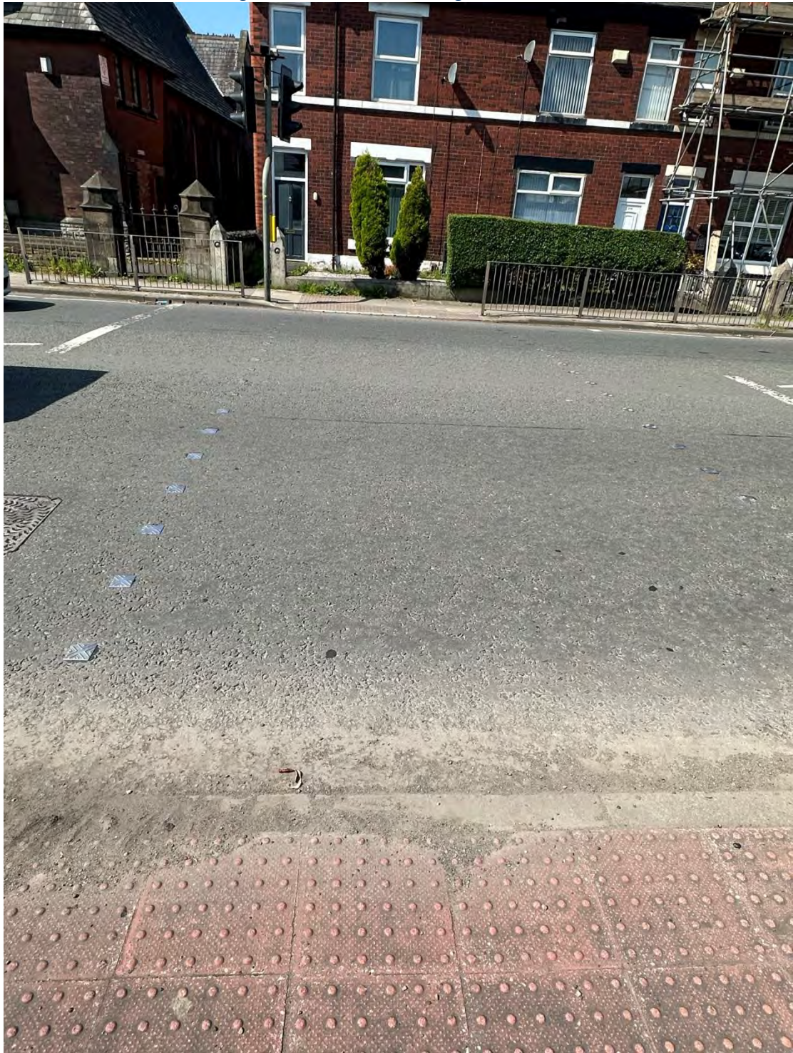
Photo 5 – Manchester Road Signalised Pedestrian Crossing
