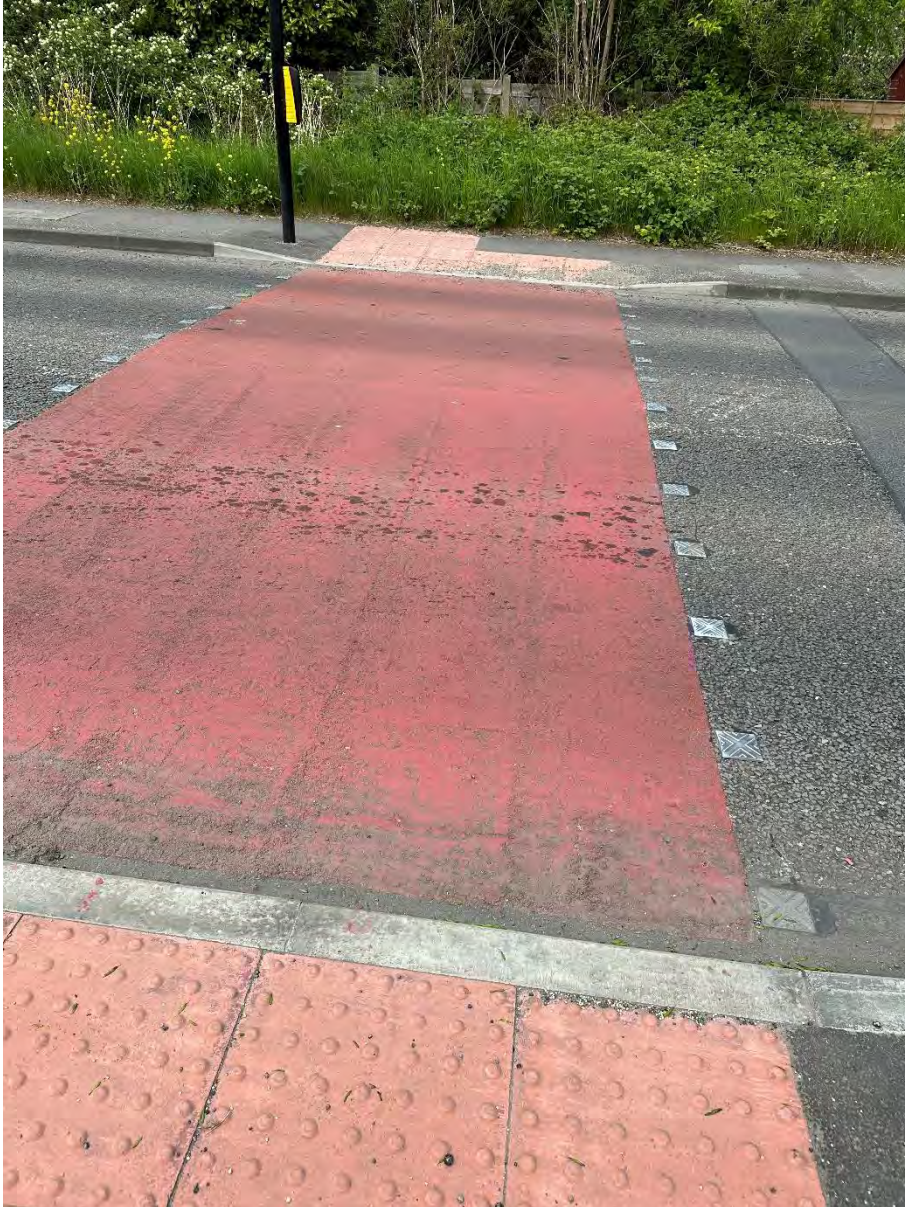
Photo 3 – Signalised Pedestrian Crossing, 350m south of the site.
