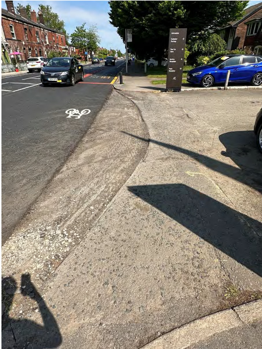
Photo 8 - Unlevelled Surfaces due to Recent Road Improvement Works
