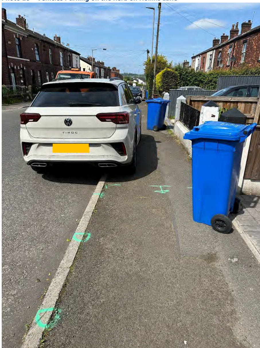
Photo 10 – Vehicles Parking on the Kerb on Hollins Lane
