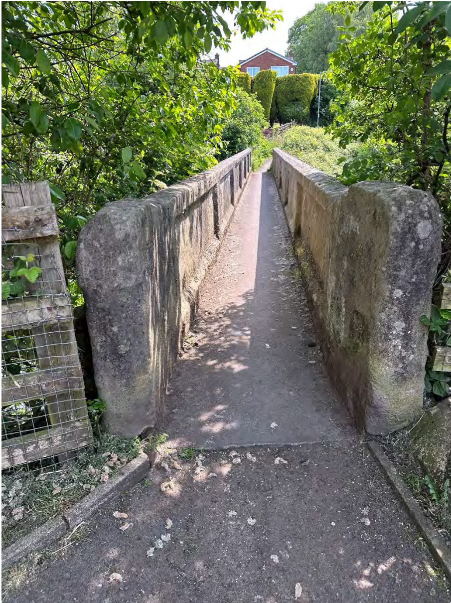
Photo 13 – Roch Valley Greenway Bridge
