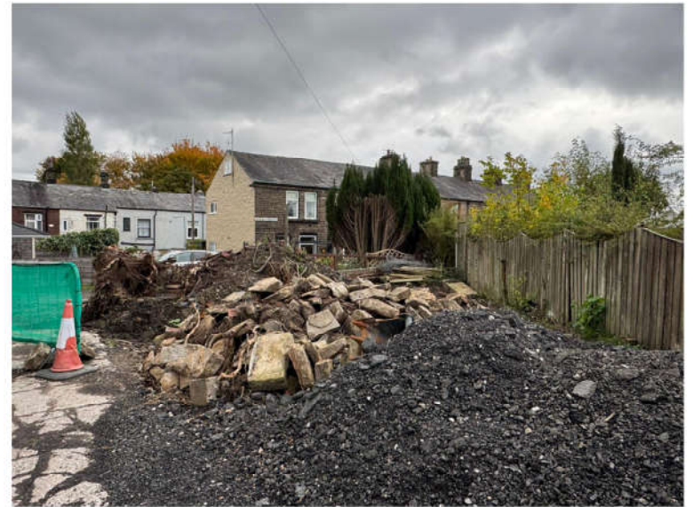
Looking southeast at stockpile
