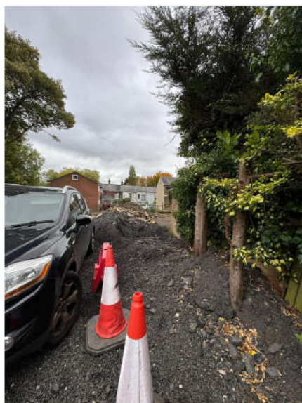
Looking east along south boundary
