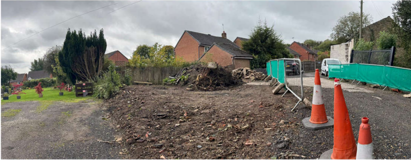
Panoramic photo looking south to west
