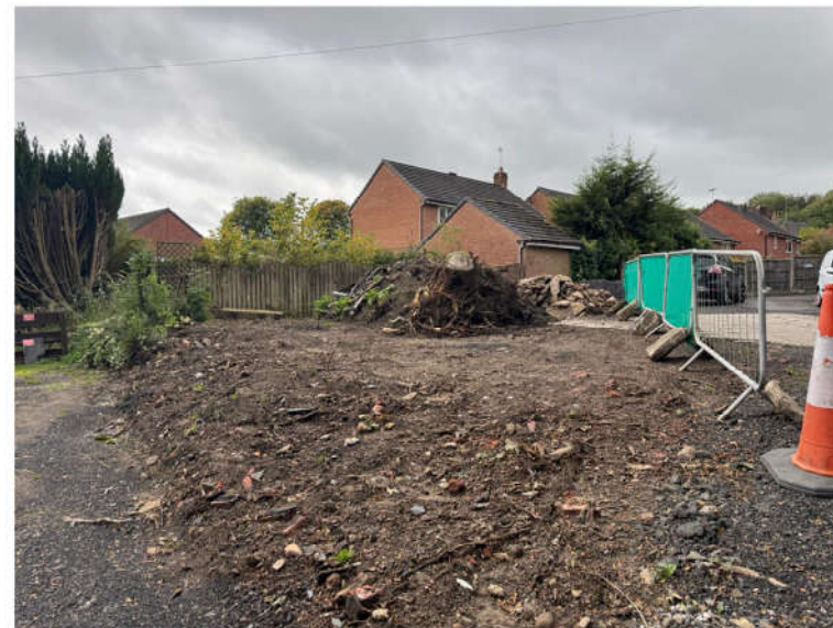
Looking southwest at made ground
