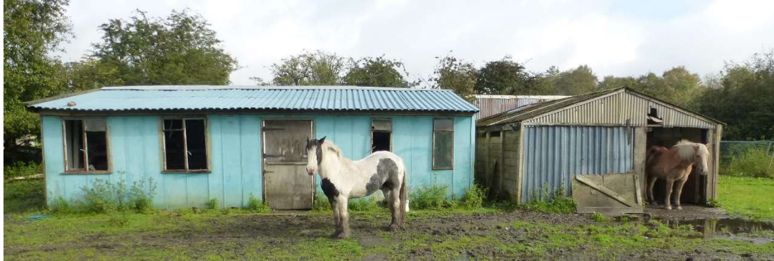
South Elevation of existing buildings.
