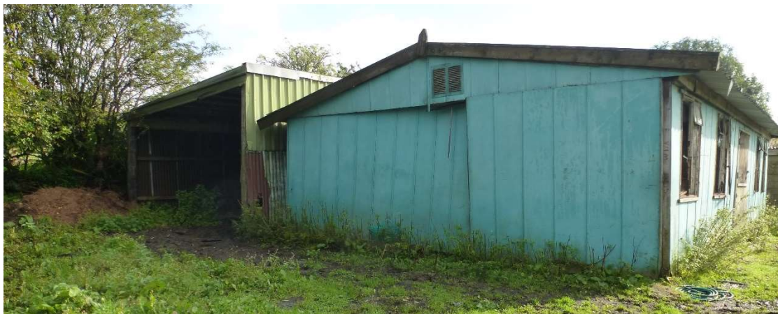
East Elevation of existing buildings.
