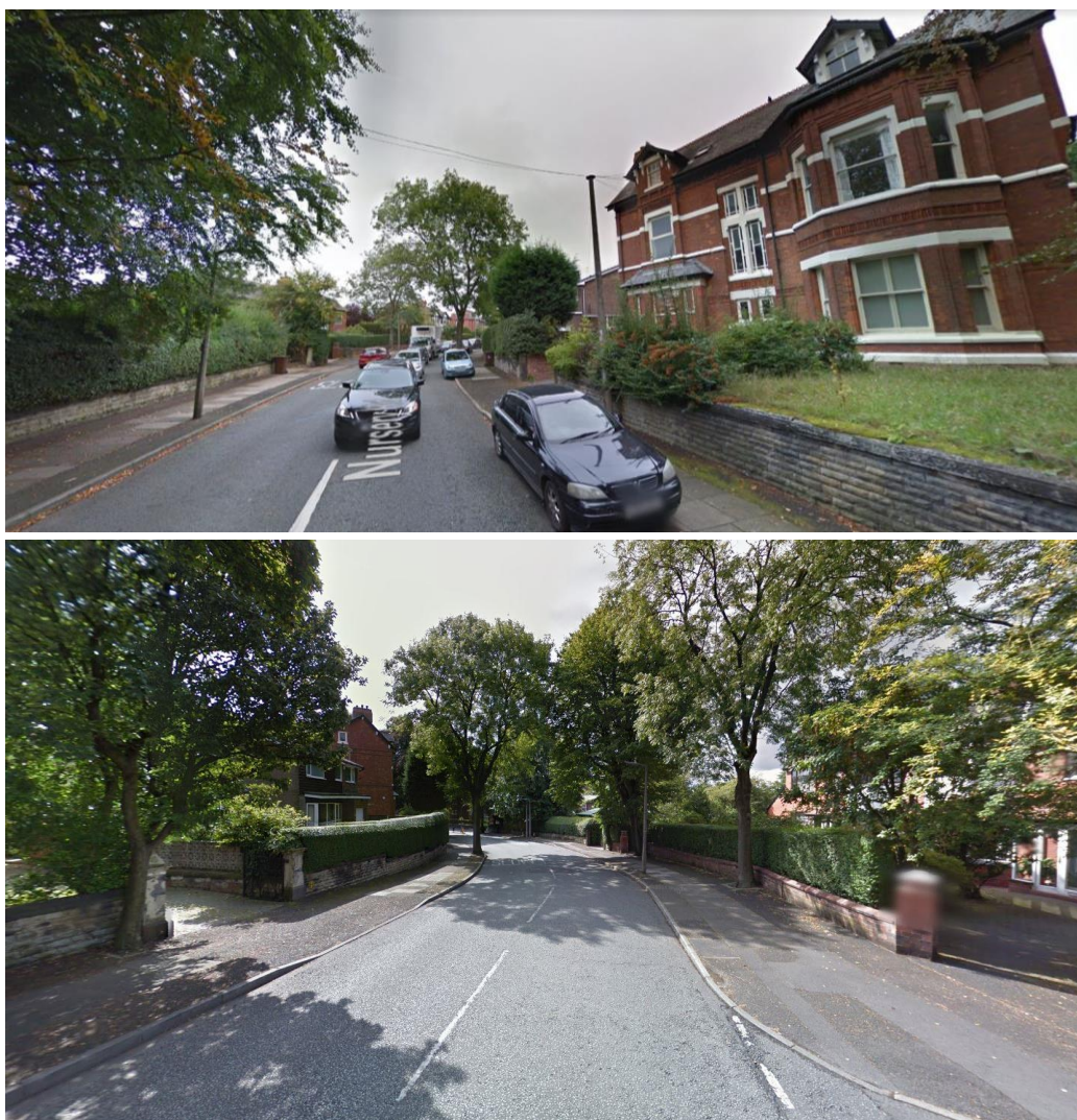
Above – views from the top and bottom of Nursery Road within the Conservation Area Boundary. Applicant property dwarfed by the neighbouring 59 Poppythorn Lane.
