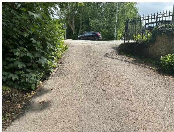
Exit of road to Hare and Hounds and traffic lights
