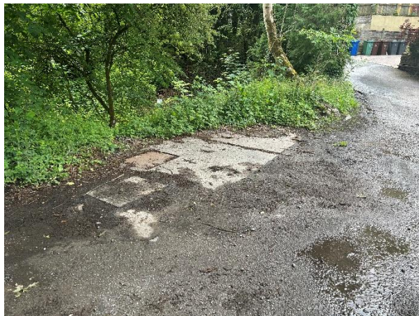
Septic tank location for Halter Inn
