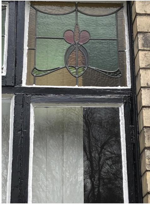
Years of paint applied to existing timber widows and bowed glass panels with broken glass
