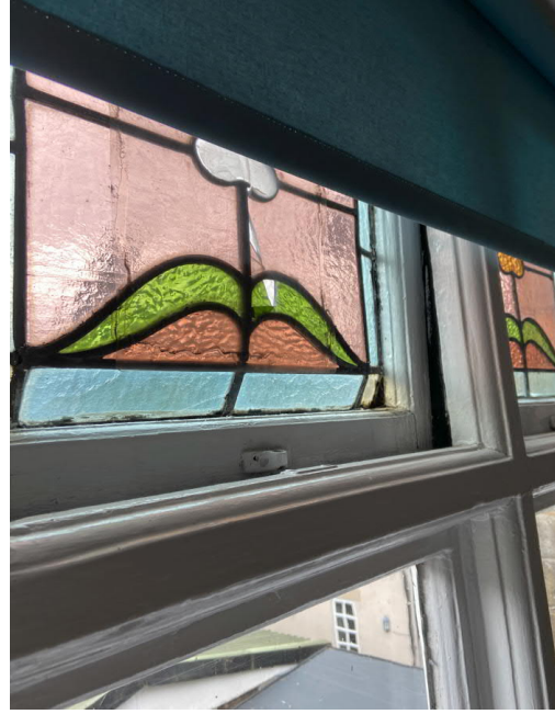
Years of paint applied to existing timber widows and bowed glass panels with broken glass
