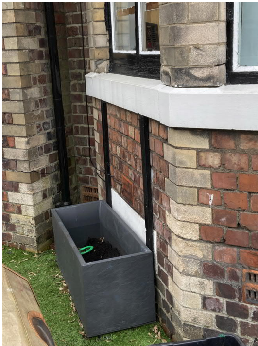
Basement windows and lightwells typically protected by planters for safety reasons And high level opening lights
