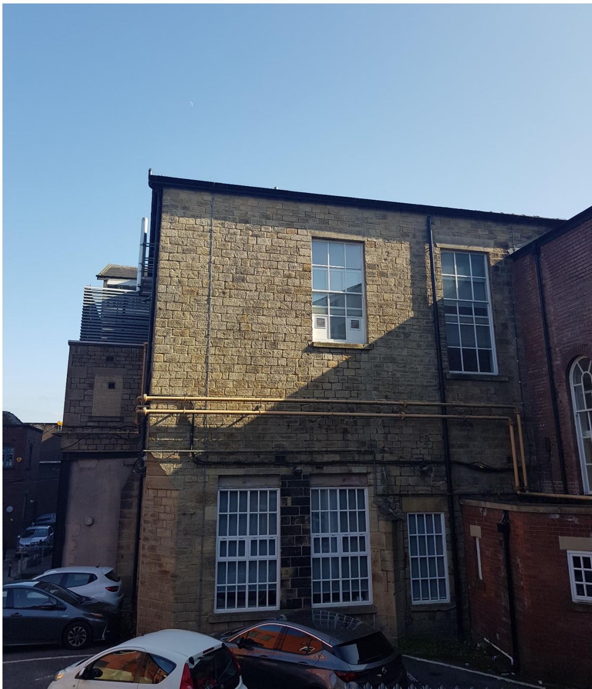
View from the rear courtyard towards the proposed placement of the solar panels
