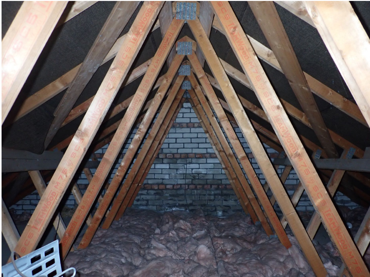
3.2a – The roof void.
