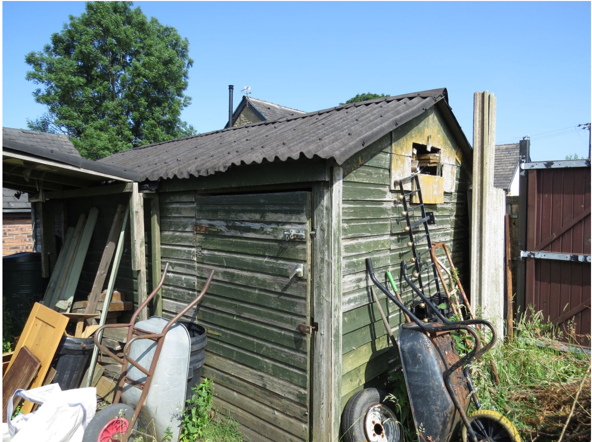
11 – The timber outbuilding has a bitumen sheet roof and single layer boarded walls.
