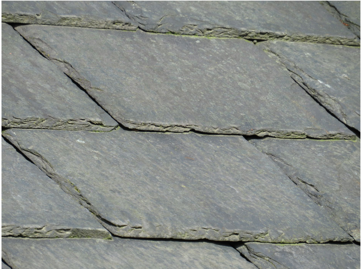
3 – Roof tiles are in good condition with no suitable gaps.
