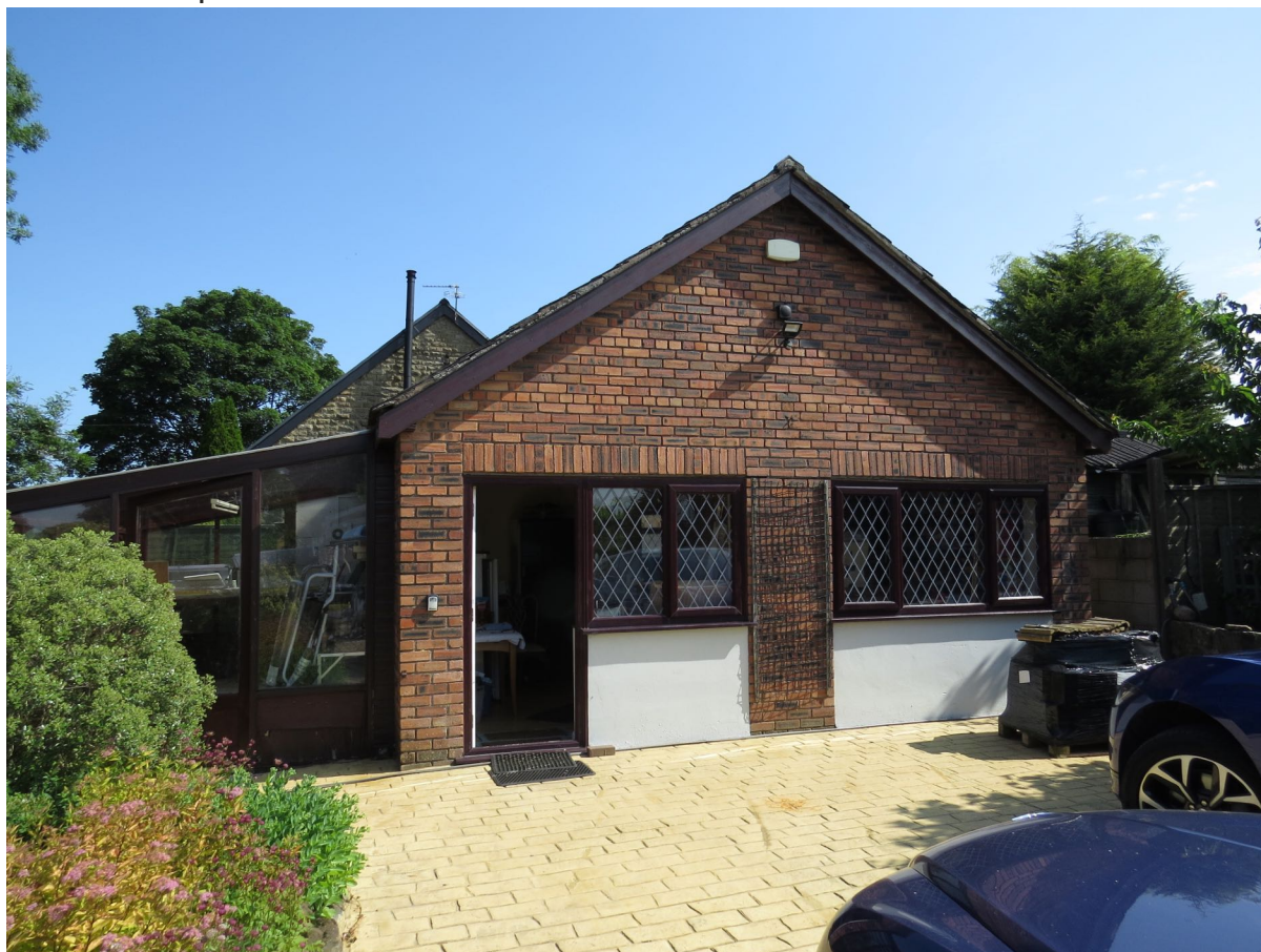
3.1a – The front of the annex.
