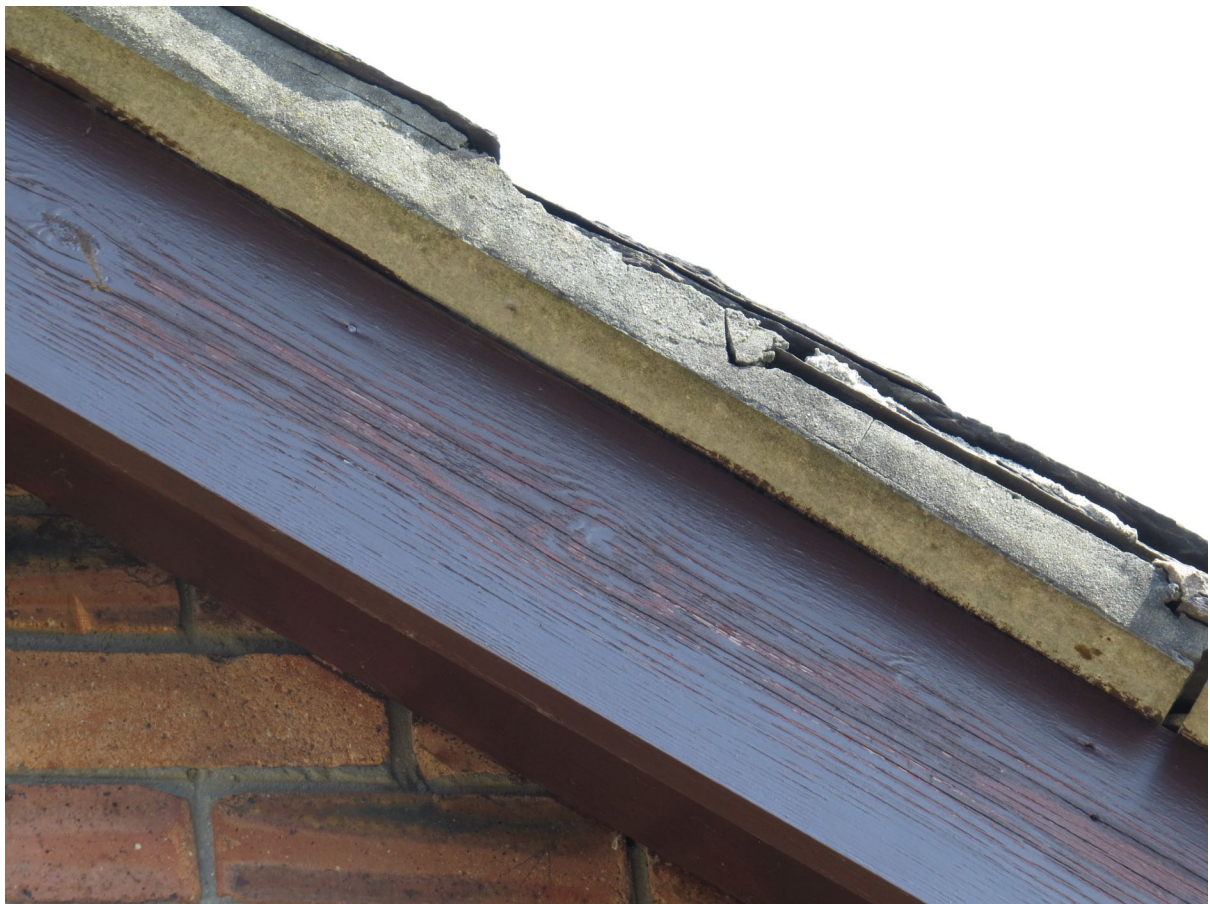
8 – Verges are sealed with cement minor gaps were checked using an endoscope.
