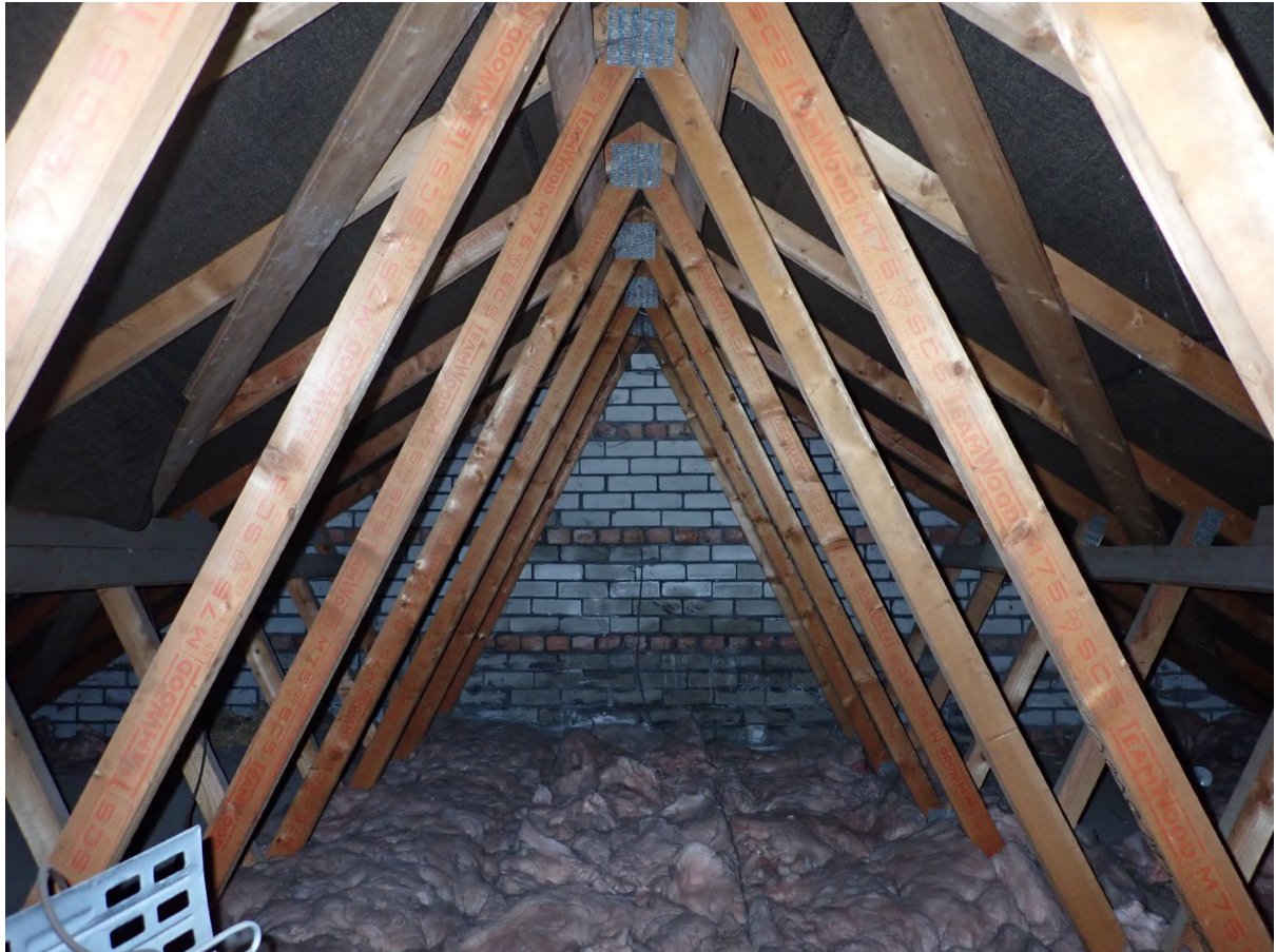
9 – The annex has a single roof void which is not used for storage.
