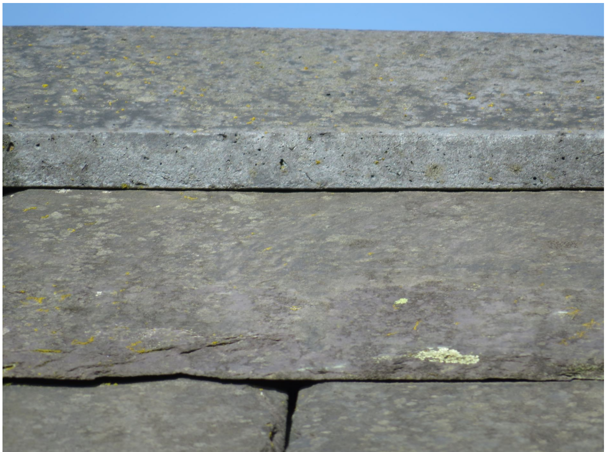
4 – Ridge tiles are laid tightly against roof tiles.
