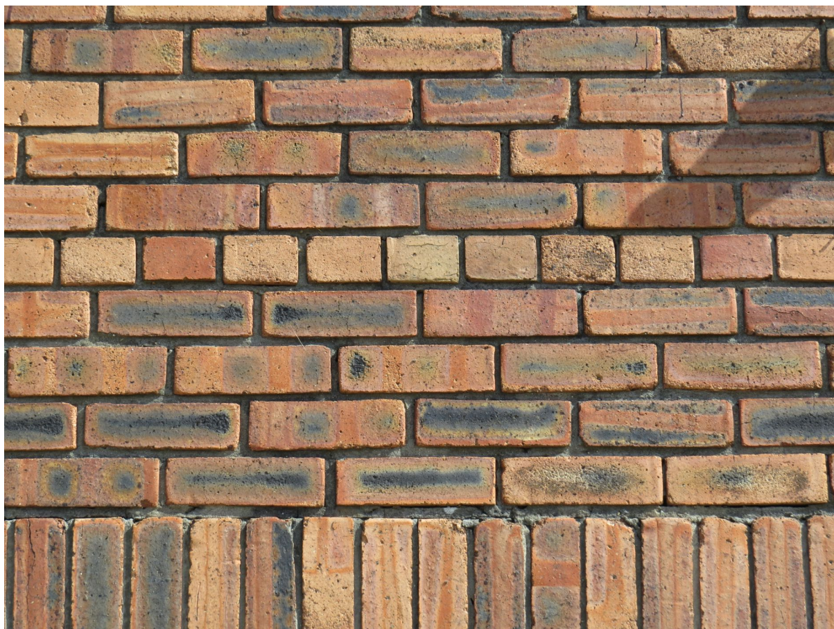
6 – Brickwork and mortar are in good condition with no suitable gaps.
