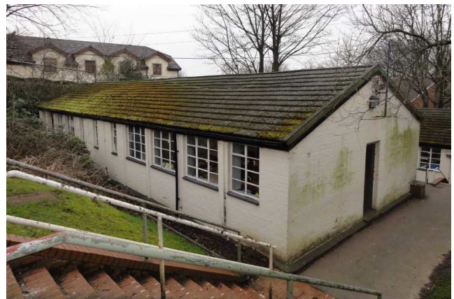
View of Temporary Building to be demolished
