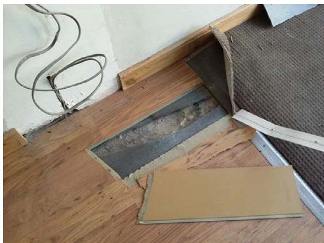
Sample No: 21/11/B/25/PK19 G.08 Shop unit Floor Bitumen adhesive No Asbestos Detected
