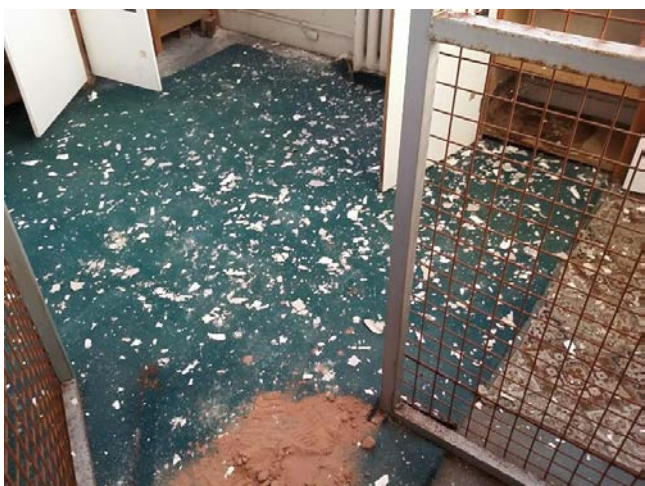
Sample No: Refer to Sample 21/11/B/25/PK5 2.10 Store Floor VFC No Asbestos Detected
