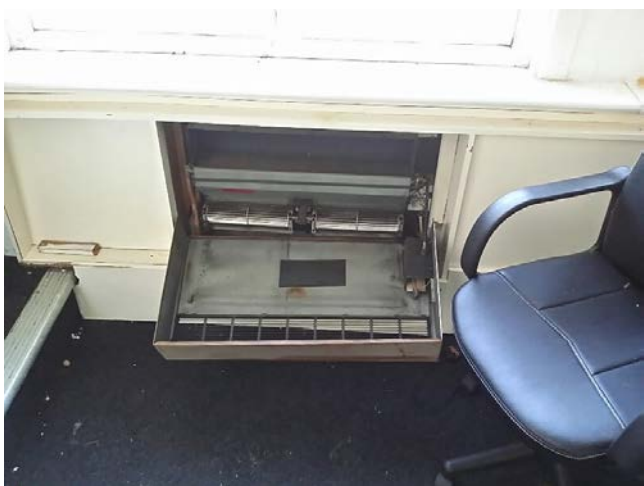
Sample No: 21/11/B/25/PK11 1.11 Store Wall behind radiator Insulation board No Asbestos Detected
