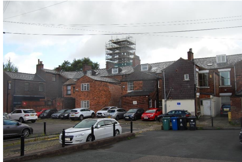
2-14 Manchester Rd from the west
