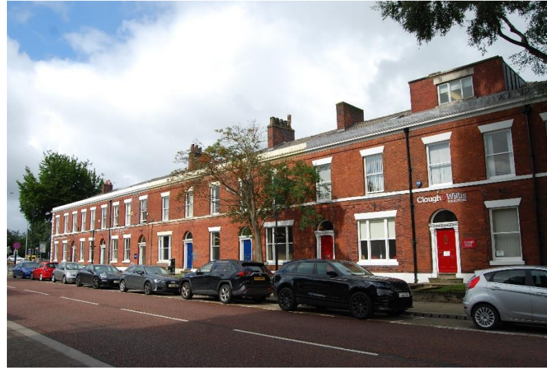
2-14 Manchester Rd from the north east
