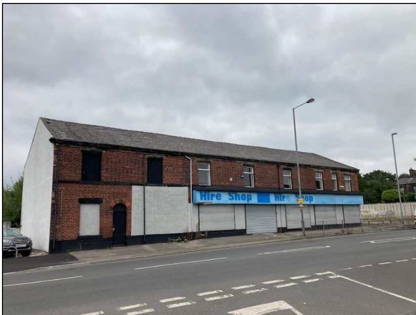
Photograph 1 showing the building
