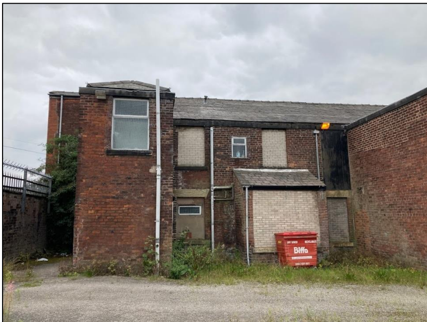
Photograph 7 showing the rear elevation of the building
