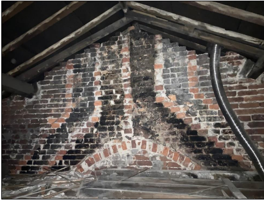
Photograph 18 showing one of the gable walls
