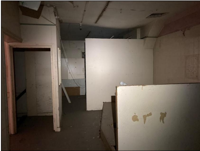
Photograph 14 showing the interior of the former commercial part of the building
