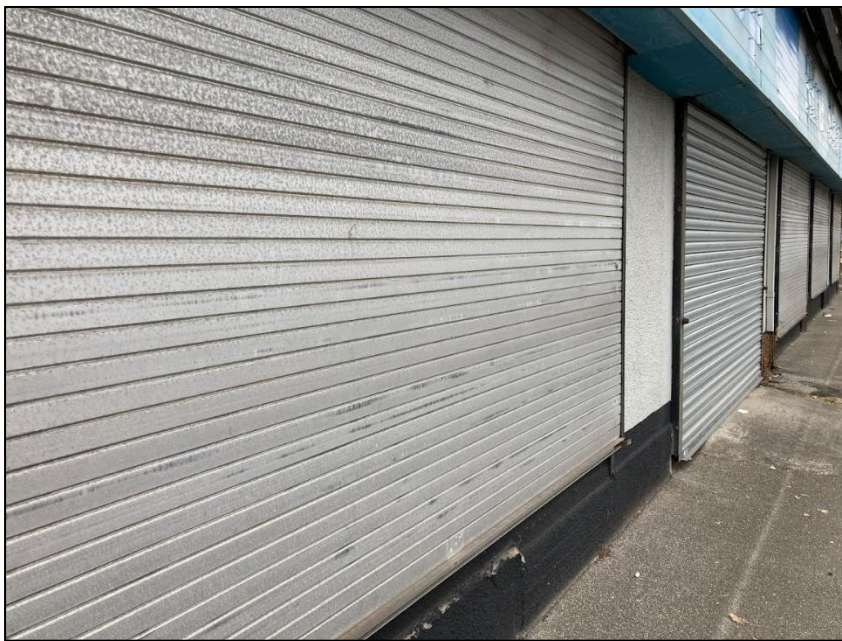
Photograph 9 showing the roller-shutters across the building's frontage
