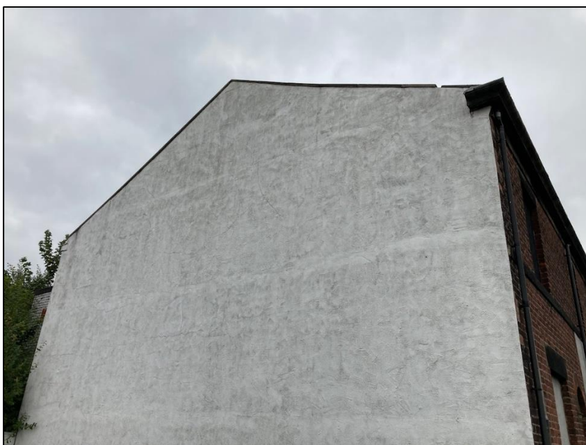
Photograph 4 showing the rendered western gable end of the building
