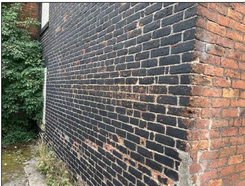
Photograph 3 showing the exterior of the building
