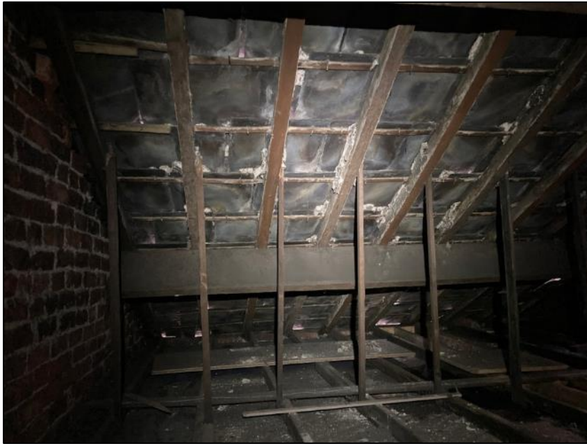
Photograph 22 showing the underside of the roof tiles
