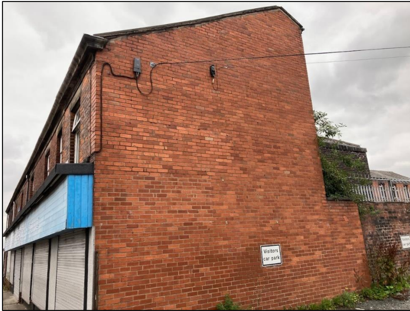
Photograph 2 showing the exterior of the building
