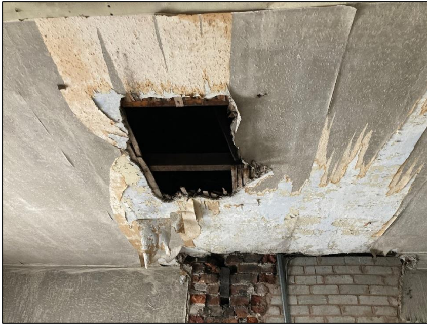
Photograph 16 showing on of the access holes in the former commercial part of the building
