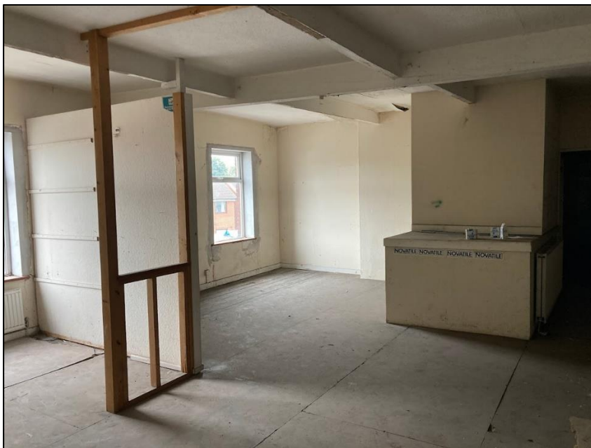
Photograph 13 showing the interior of the former commercial part of the building
