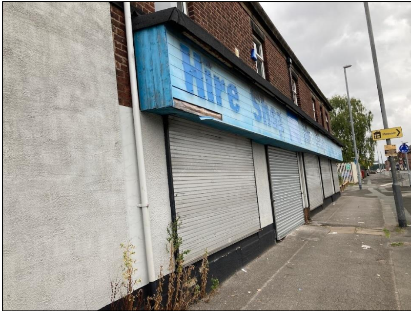
Photograph 6 showing the timber clad box feature on the building's frontage
