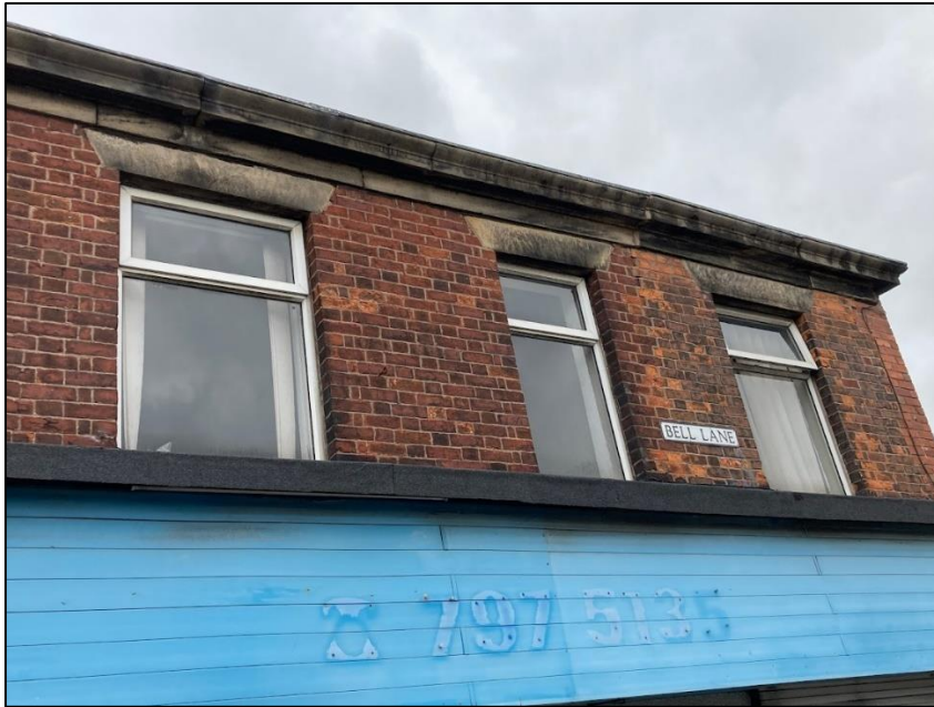
Photograph 8 showing some of the uPVC window frames
