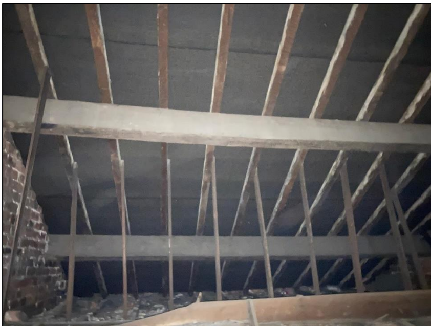
Photograph 19 showing the underside of the roof
