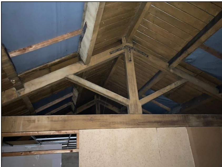
Photograph 17 showing on of the extended section of the former commercial part of the building
