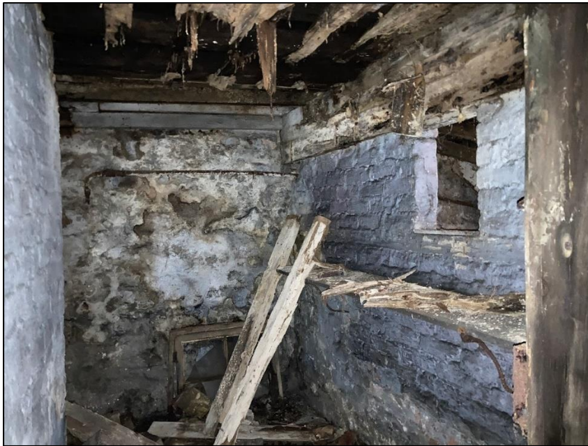
Photograph 20 showing part of the basement level
