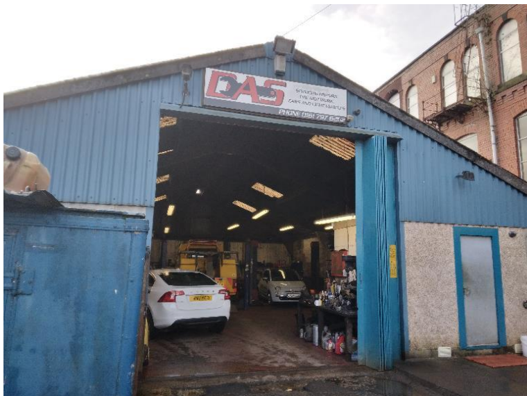
North elevation of the building
