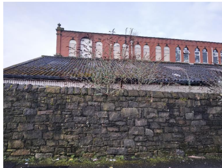
East elevation of the building (only partially visible in the photo behind an adjacent tall stone wall with buddleia growing out of it)
