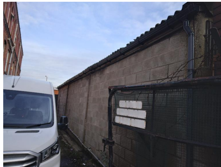
West elevation of the building
