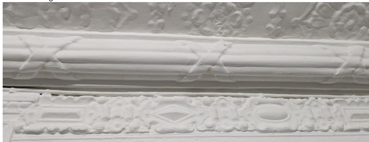
The decorative plaster at the top of the wall/bottom of the ceiling.
