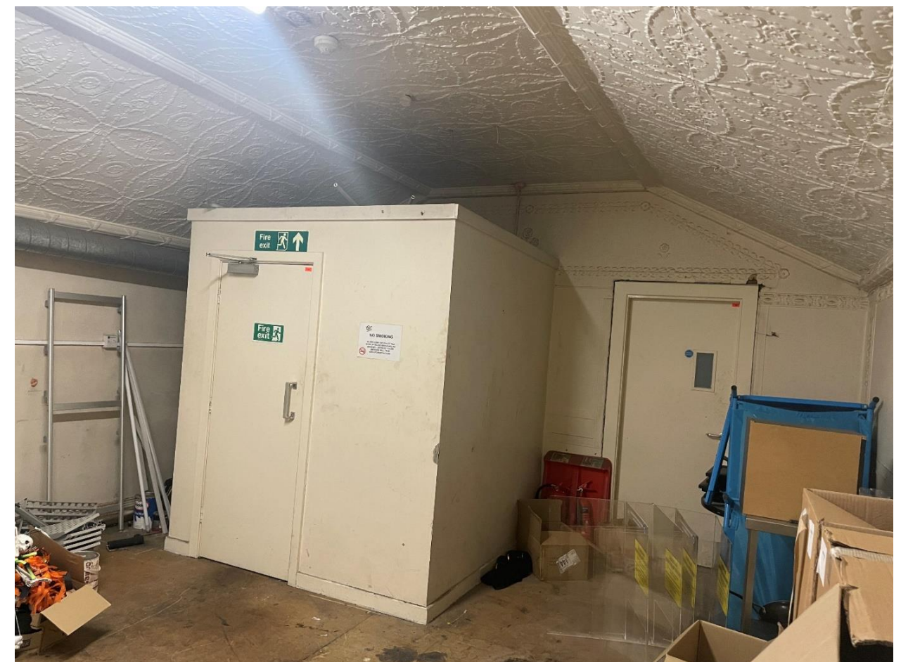
The undeveloped room on the first floor, including the lobby to be demolished and the ceiling and end wall with historic decorative plasterwork.
