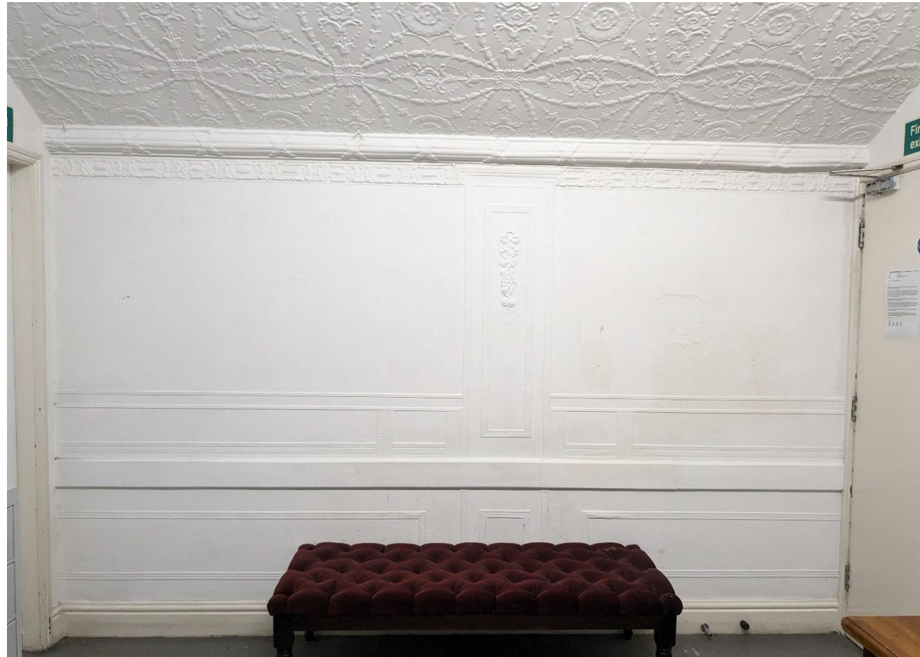
The historic plasterwork in the existing staff room.
