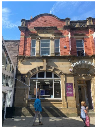
Window A. Modified to form larger glazed opening.
