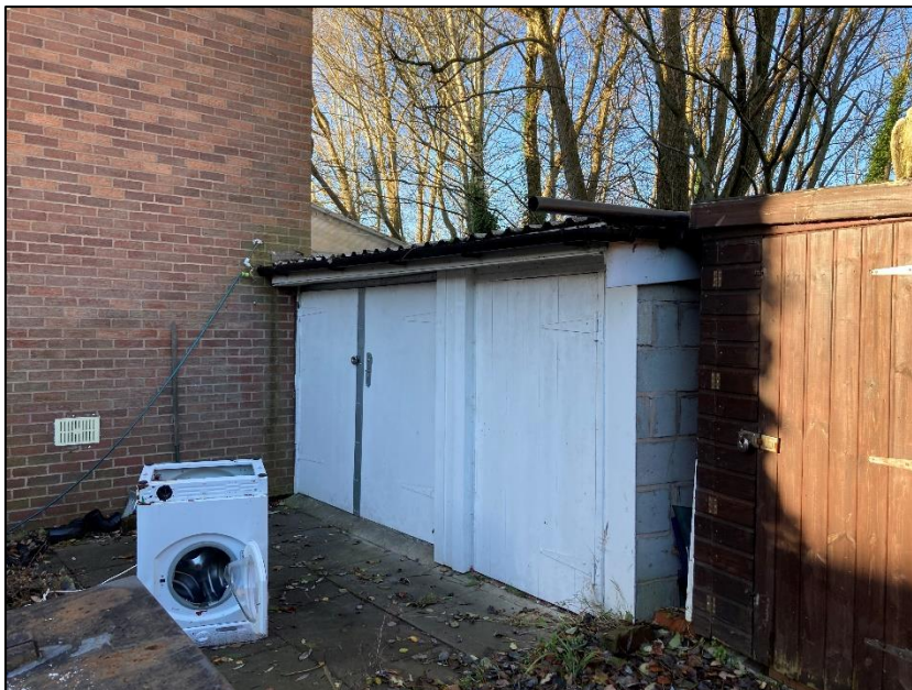
Photograph 6 showing the garage
