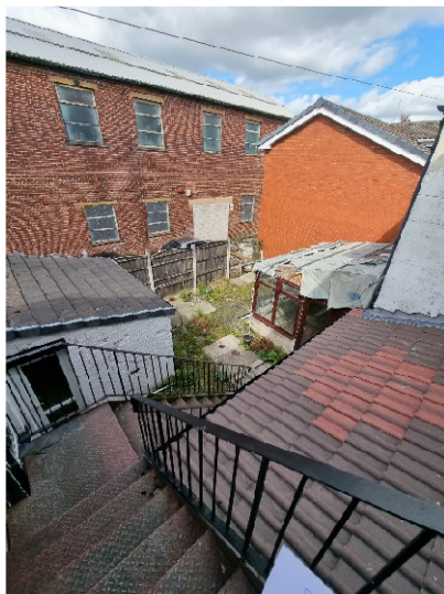
Fig 5– Rear staircase and yard
