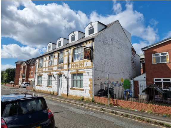
Fig 1 – View of front of property
