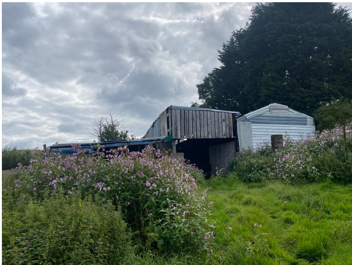
Proposed removal of existing agricultural buildings (above)
