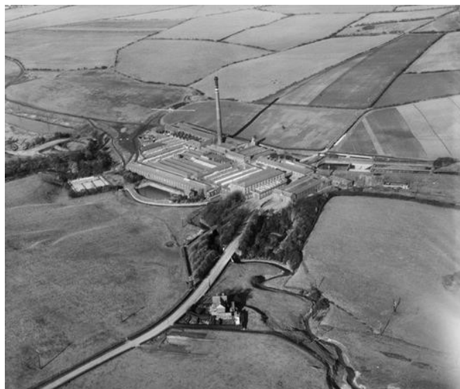
Figure 2 – Pilsworth Bleach Works © Britain from Above
