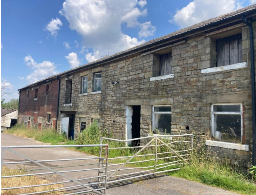
Figure 7 – Front Elevation of the Barn & Stables © Laith Heritage
