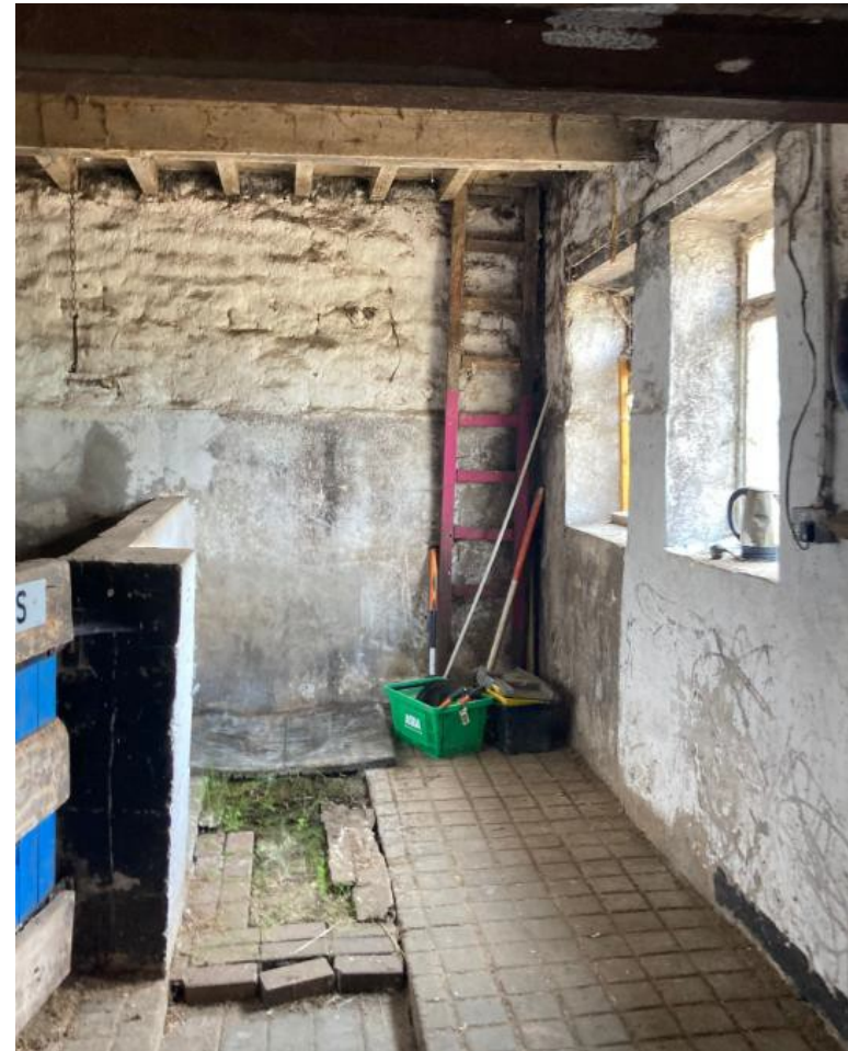
Figure 8 – Barn interior © Laith Heritage
