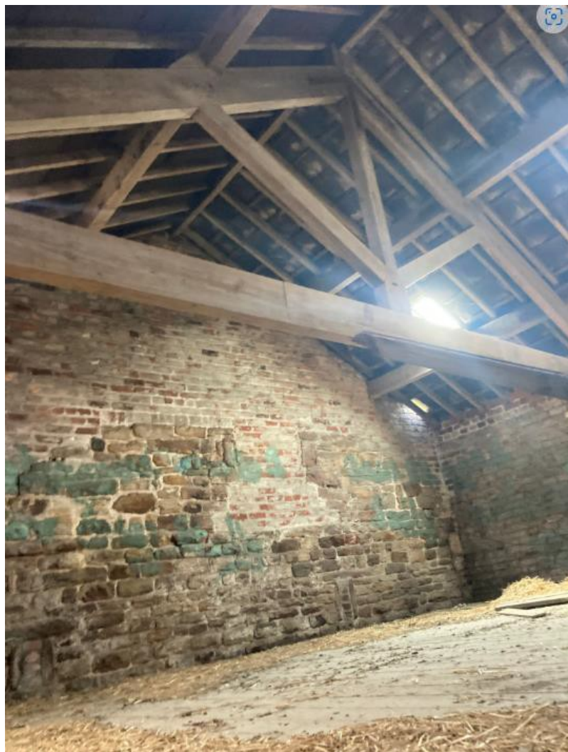
Figure 12 – Example of the king post trusses found on site © Laith Heritage
