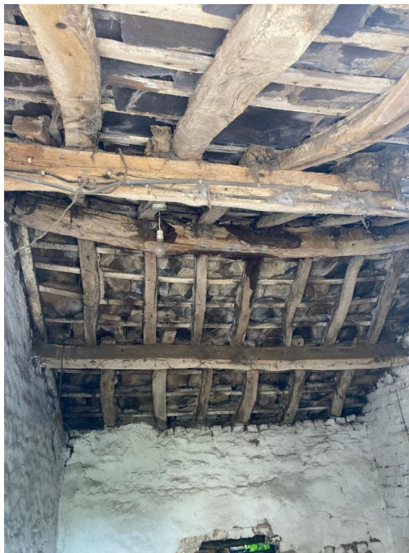
Figure 13 – Timber beams & purlins in animal shelter © Laith Heritage
