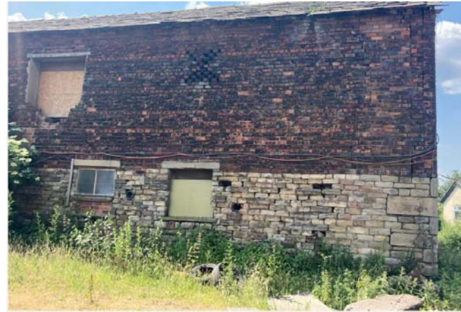
Figure 10 – Rear Elevation of the Stables © Laith
