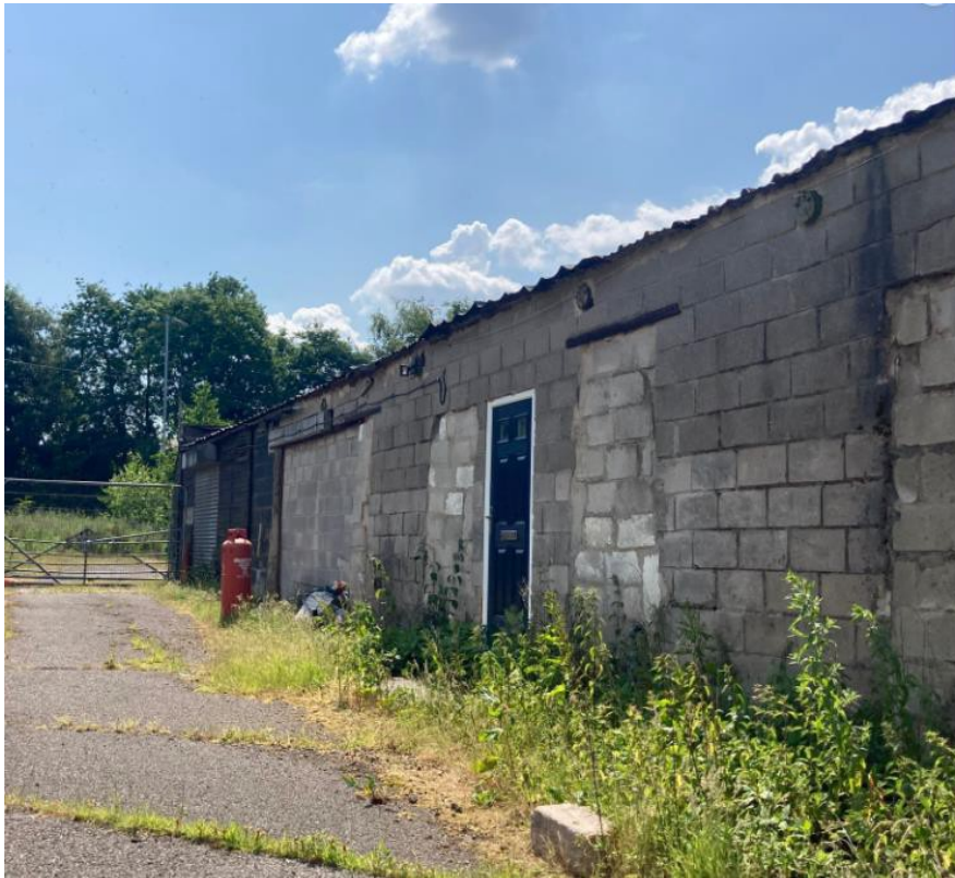
Figure 9 – Rear Elevation of the Barn © Laith Heritage
