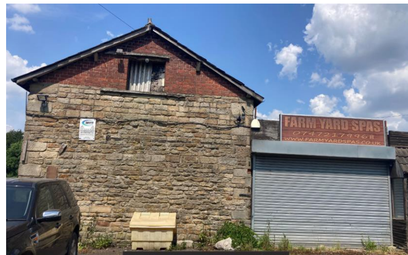
Figure 6 – Southern Elevation of the Barn © Laith Heritage
