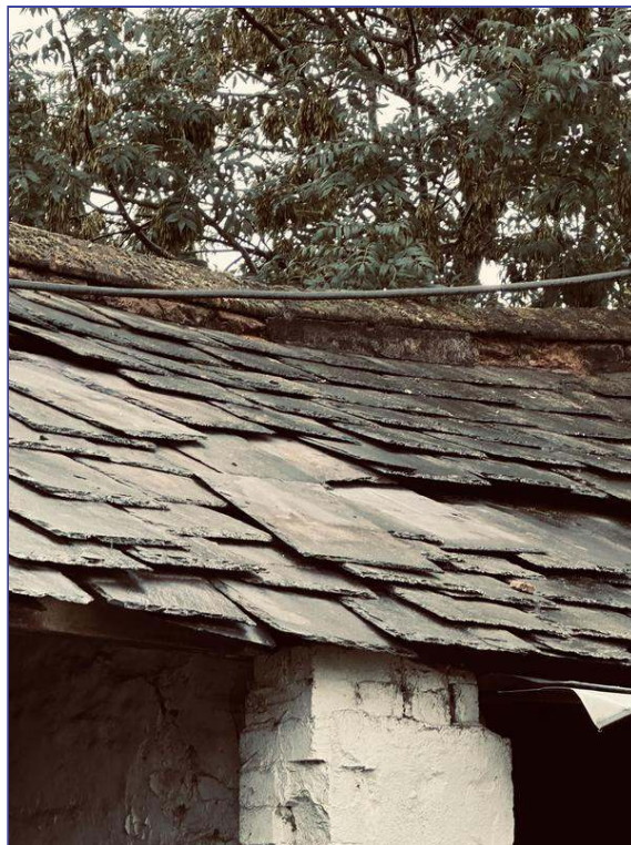
Photo 3 - Slates to be taken down carefully to reduce breakage.
