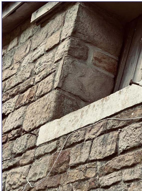
Photo 61 - Wall thickness 400 mm
