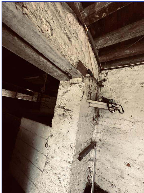
Photo 41 - All internal lintels to be checked closely.
