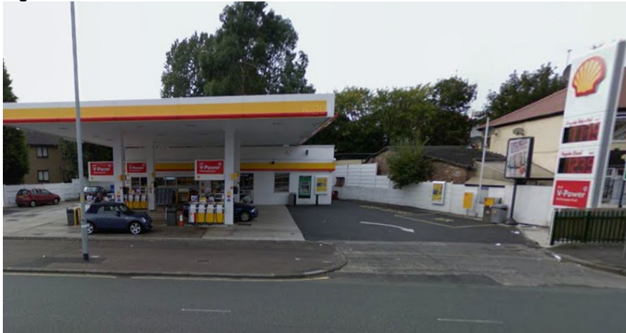
Figure 1: View of the site
