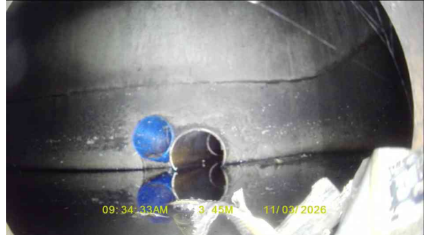
2, 00:00:23, 3.45 m Finish node, manhole, reference: MH05
