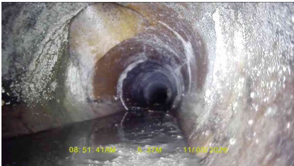
3, 00:00:32, 5.37 m Junction at 10 o'clock, 150mm dia
