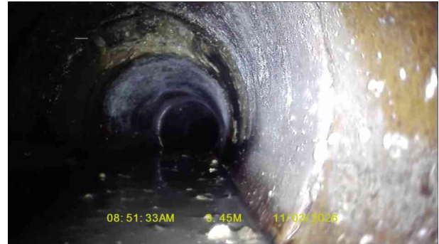
2, 00:00:24, 3.45 m Junction at 12 o'clock, 150mm dia
