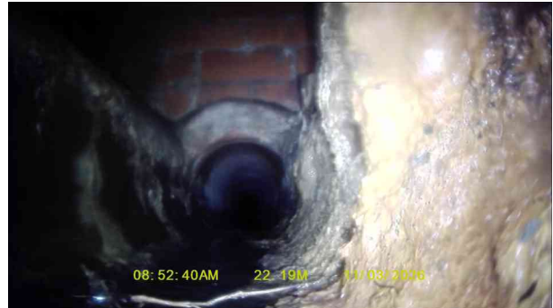
6, 00:01:31, 22.19 m Finish node, manhole, reference: MH02
