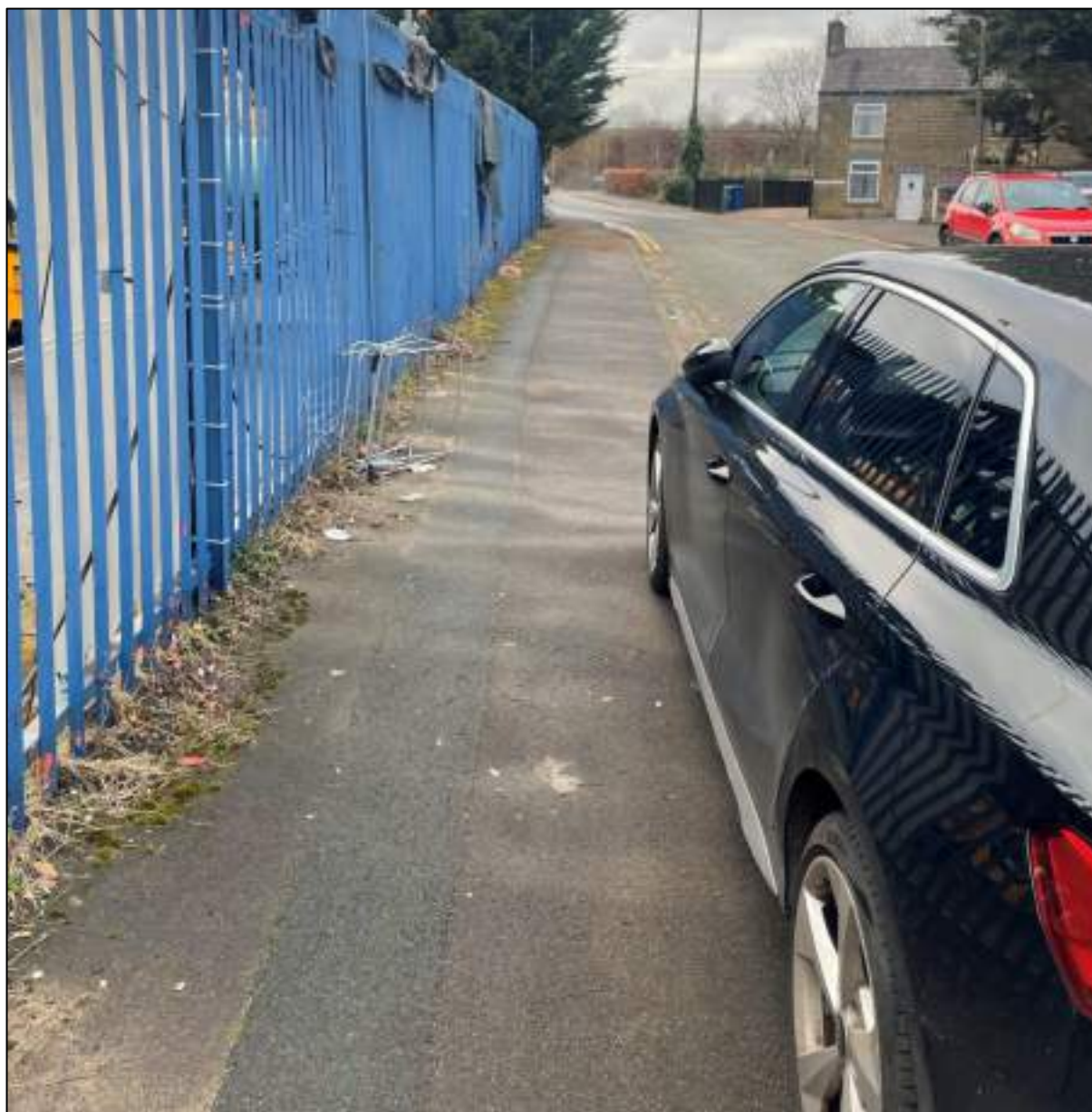
213m – Utilities reinstatement in the footpath
