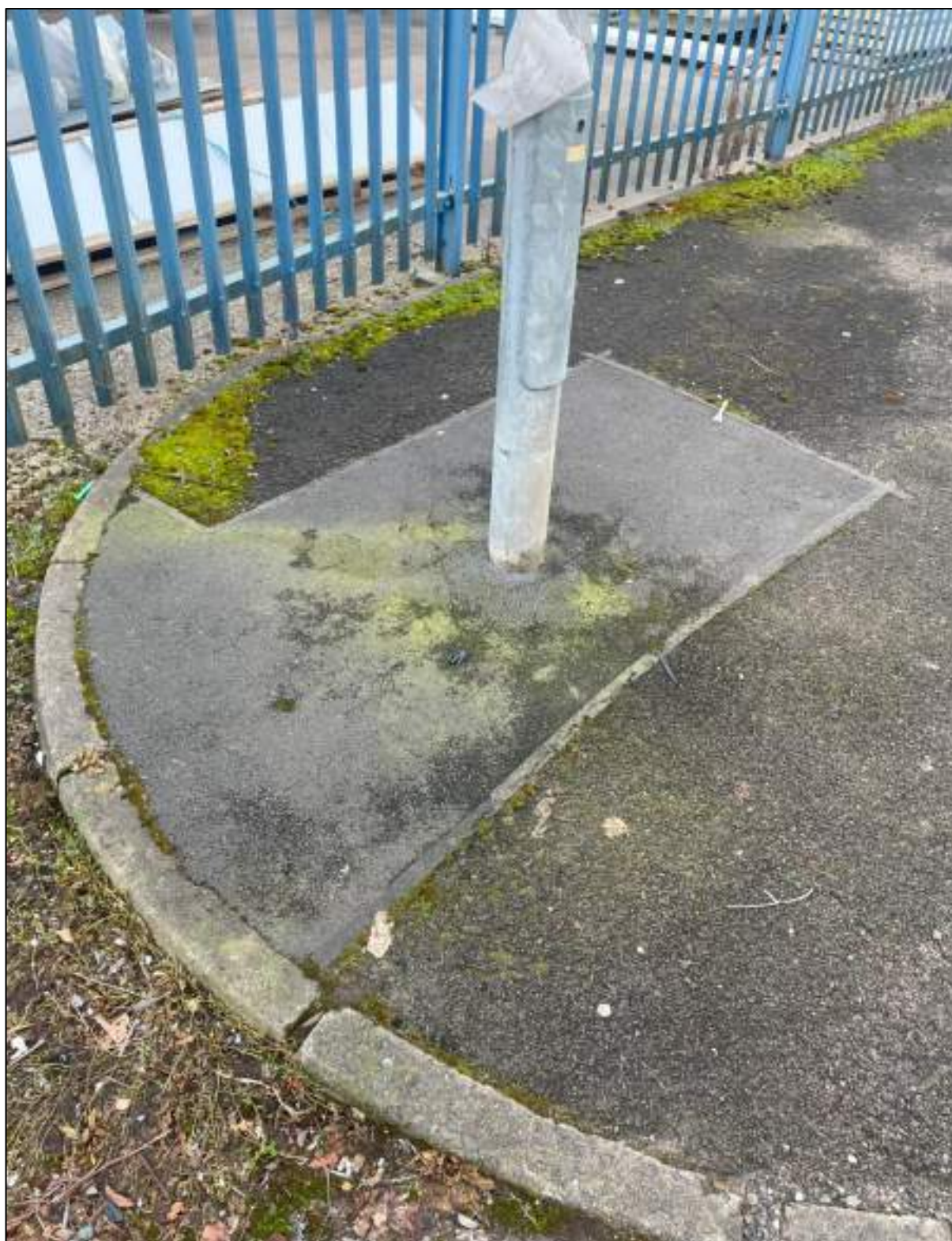
147m - Lamppost with reinstatement at base.
