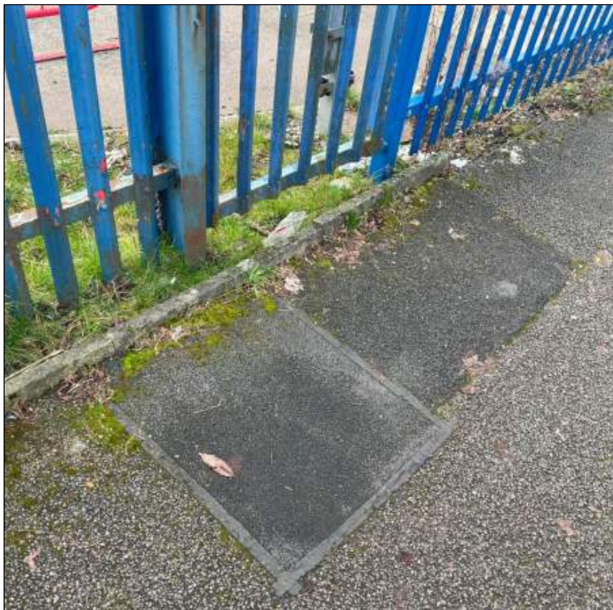
20m - Patching of footway.
