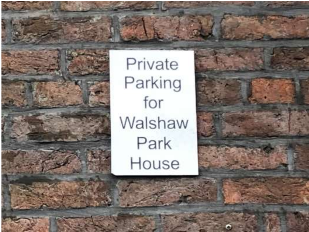
Image 7 – Car parking signage to side elevation
