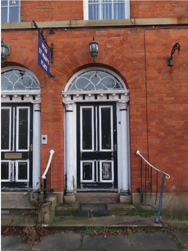
Repair to original balustrade to number 18.
