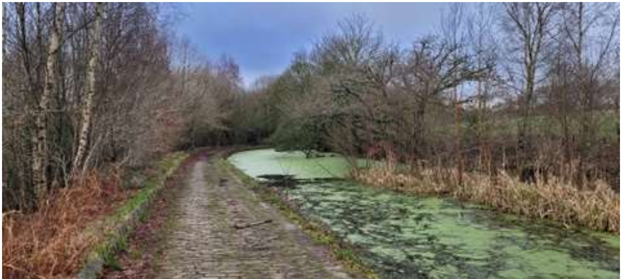
Photo 14 – Further Example of Canal Condition
