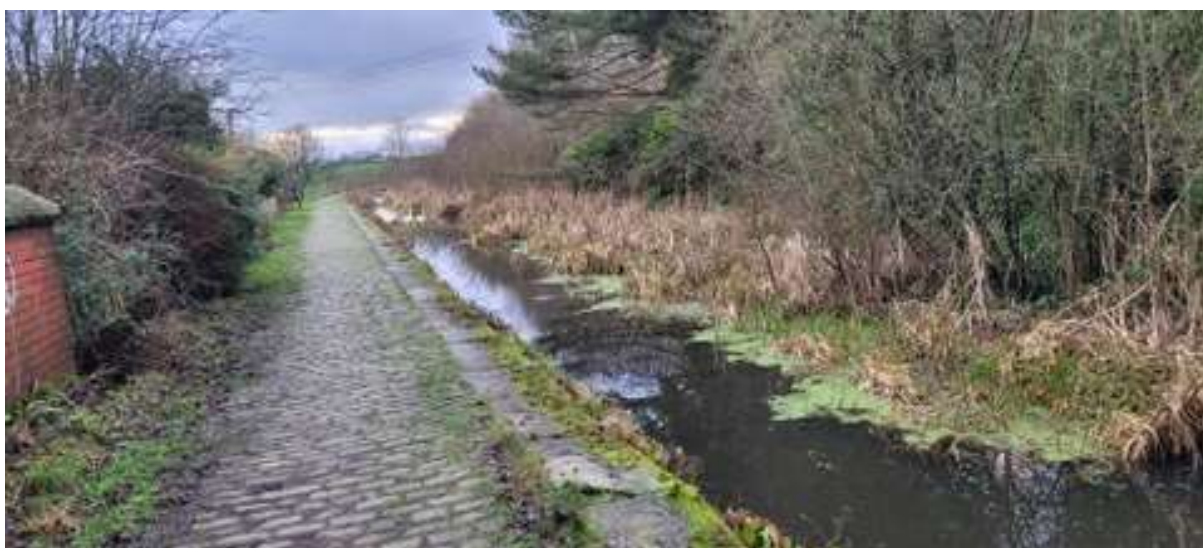
Photo 12 – Example of canal overgrown with weeds
