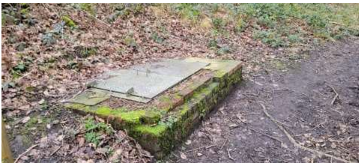
Photo 17 – Manhole Adjacent 1932 Breach, indicates diversion into river Irwell, approx.
