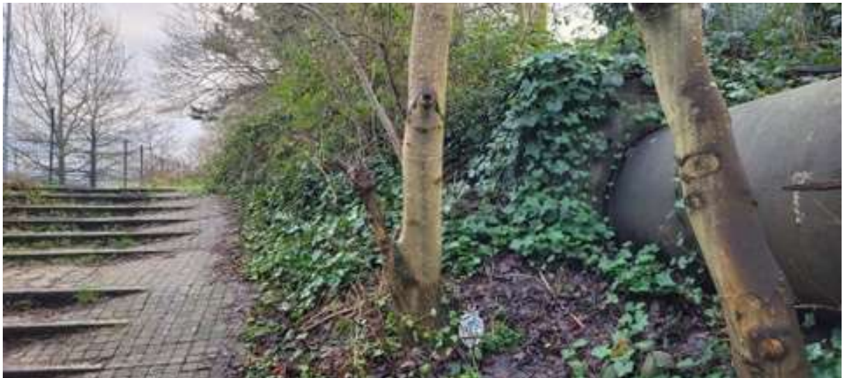
Photo 6 – Pipe interface, note steps and site boundary fence visible to left
