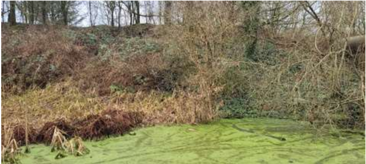
Photo 9 – General photo of Canal Bank
