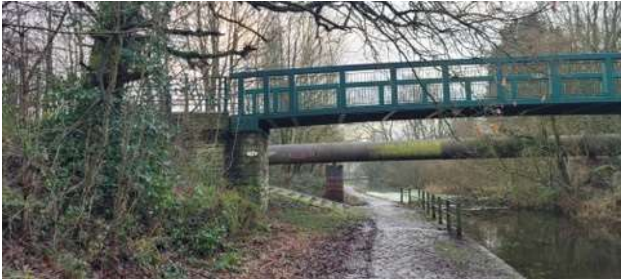
Photo 5 - Adjacent site, Note foot bridge and steel pipe
