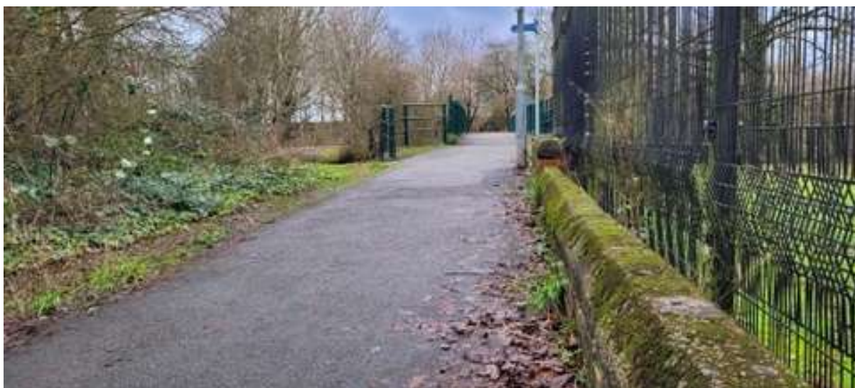
Photo 7 - Raised Footpath adjacent to site boundary, note bridge and pipe crossing canal
