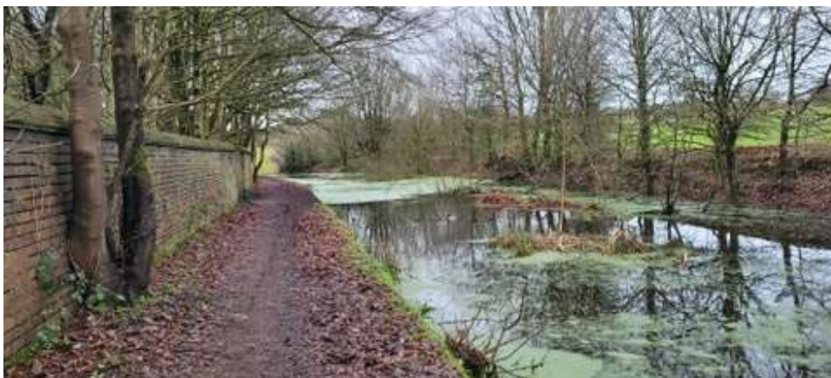
Photo 15 – Further Example of Canal Condition
