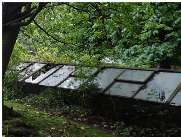
Photo 12: Building 1, adjacent to the eastern site boundary
