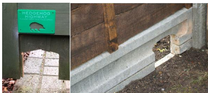
Insert 5: Showing wildlife access gap within fencing
