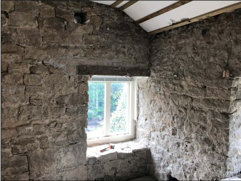
5.8 Natural stone faces of external walls generally dry with no major water ingress above ground.
