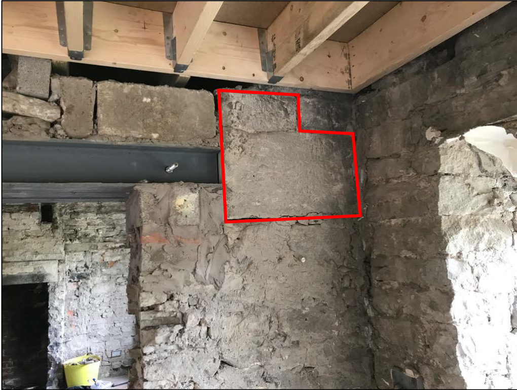
5.6 Proposed exposed stone section to remain visible within former external wall of c. 1739.
