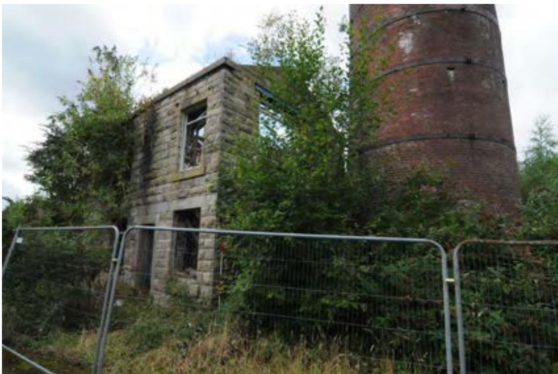
Photograph No : 61 Digital Ref: HOMI_HBR_0004 Direction: SW Description: East and north elevations of Building C and Chimney base
