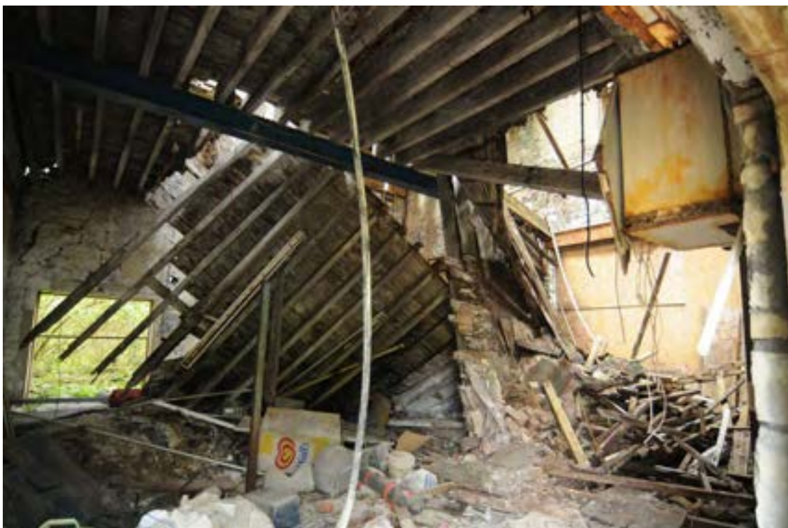
Photograph No : 53 Digital Ref: HOMI_HBR_0049 Direction: SW Description: General southern view of ground floor internal area of Building B
