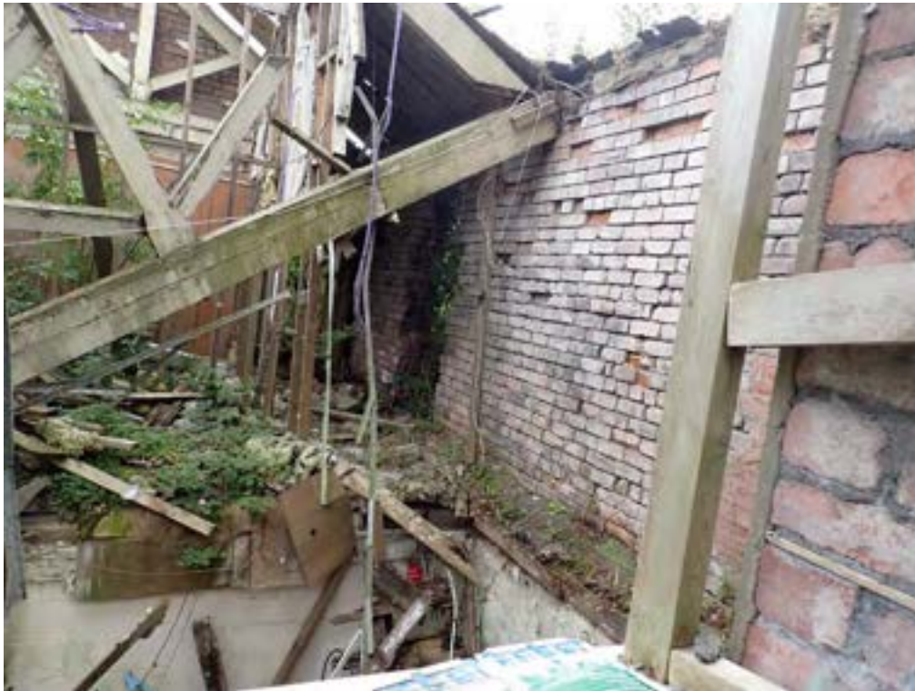
Photograph No : 83 Digital Ref: HOMI_HBR_0094 Direction: SW Description: King post trusses and general view of first floor of Building C
