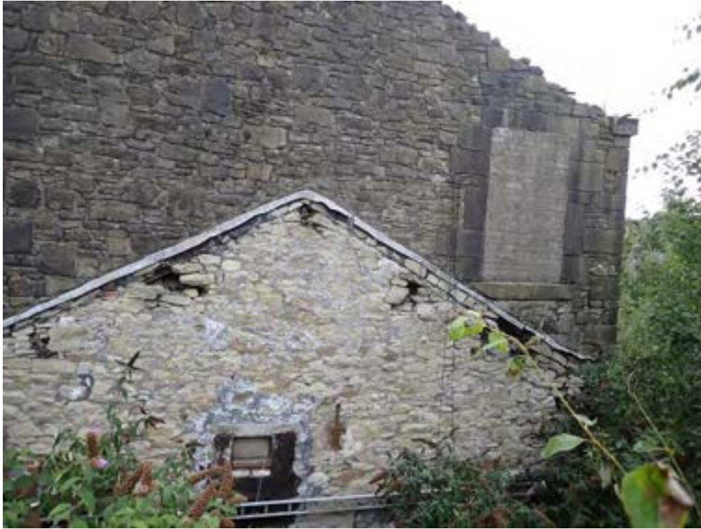
Photograph No : 33 Digital Ref: HOMI_HBR_0101 Direction: NE Description: South gable of Building B with blocked fenestration at the first floor, gable scar of former building, bearing box
