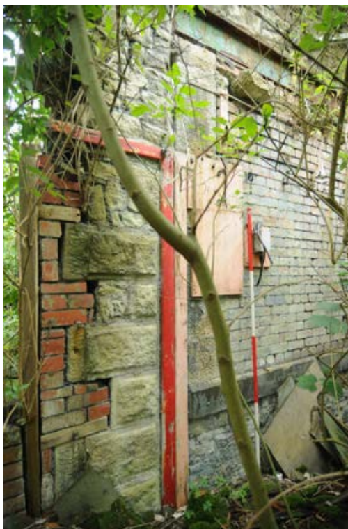
Photograph No : 30 Digital Ref: HOMI_HBR_0117 Direction: NW Description: Southern extent of east elevation of Building B with quoins at extent
