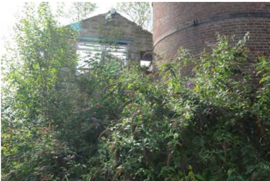
Photograph No : 63 Digital Ref: HOMI_HBR_0025 Direction: SW Description: North gable of Building C with Chimney base at NW (right)
