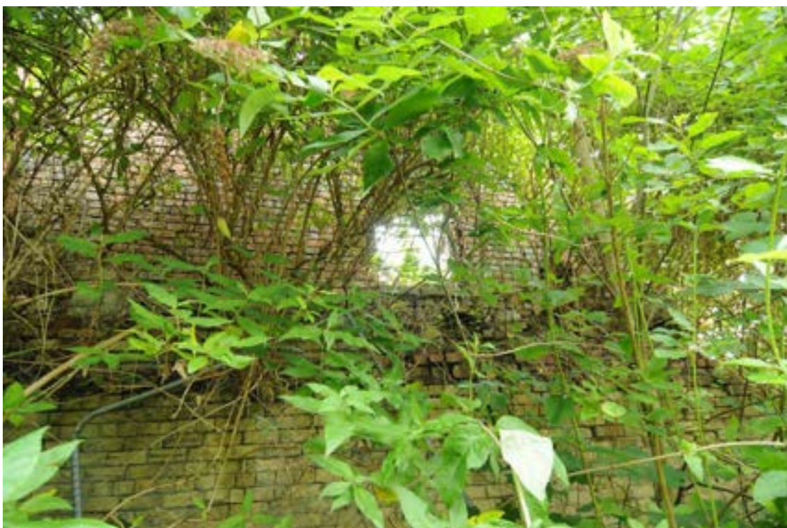
Photograph No : 86 Digital Ref: HOMI_HBR_0037 Direction: E Description: Window in first floor of west elevation of Building C, brick wall on ground floor
