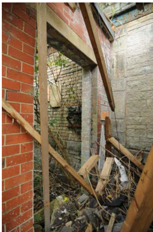
Photograph No : 49 Digital Ref: HOMI_HBR_0115 Direction: SW Description: Blocked fenestration in west elevation of Building B and general internal view of ground floor area of addition
