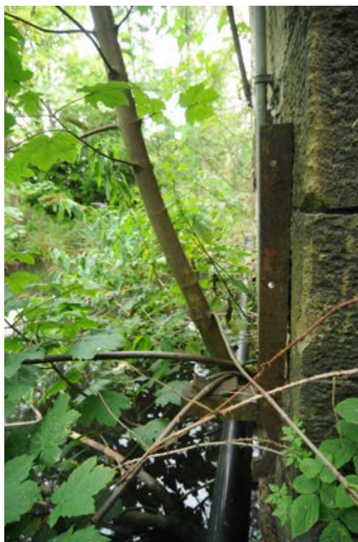
Photograph No : 45 Digital Ref: HOMI_HBR_0132 Direction: N Description: Metal fittings in southern extent of west wall of Building B
