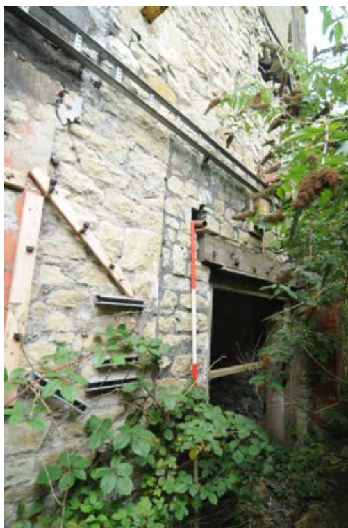
Photograph No : 38 Digital Ref: HOMI_HBR_0121 Direction: NE Description: Straight joint and change of stone at eastern side of south gable of Building B
