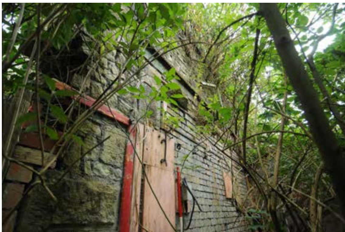
Photograph No : 50 Digital Ref: HOMI_HBR_0118 Direction: NW Description: Blocked fenestration in southern extent of east elevation of Building B with quoins at extent
