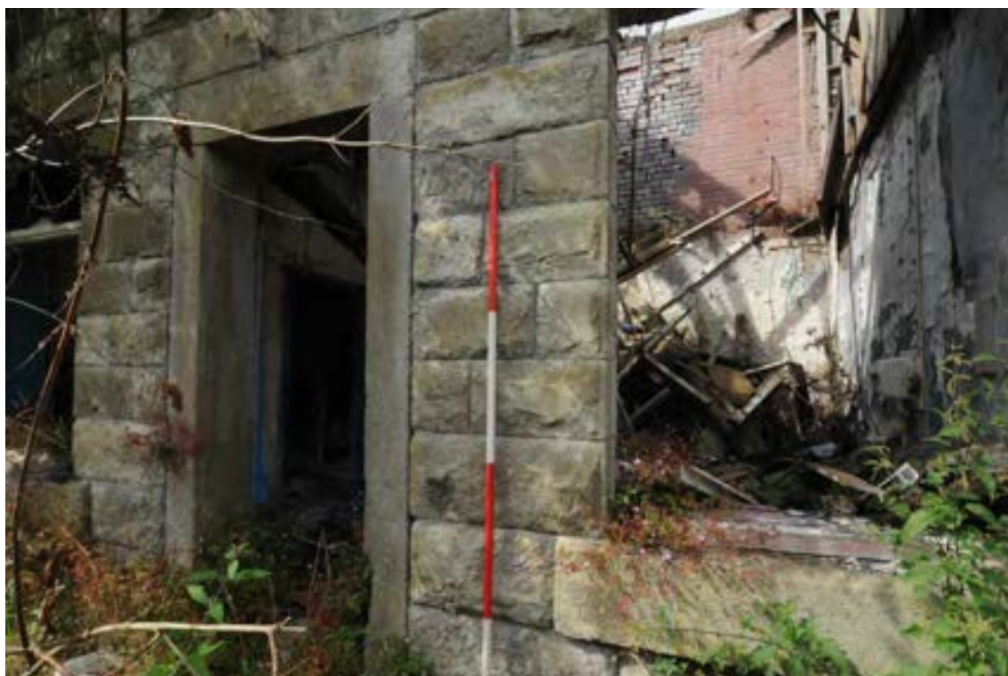
Photograph No : 70 Digital Ref: HOMI_HBR_0014 Direction: SW Description: SW view of east elevation of Building C and view into building
