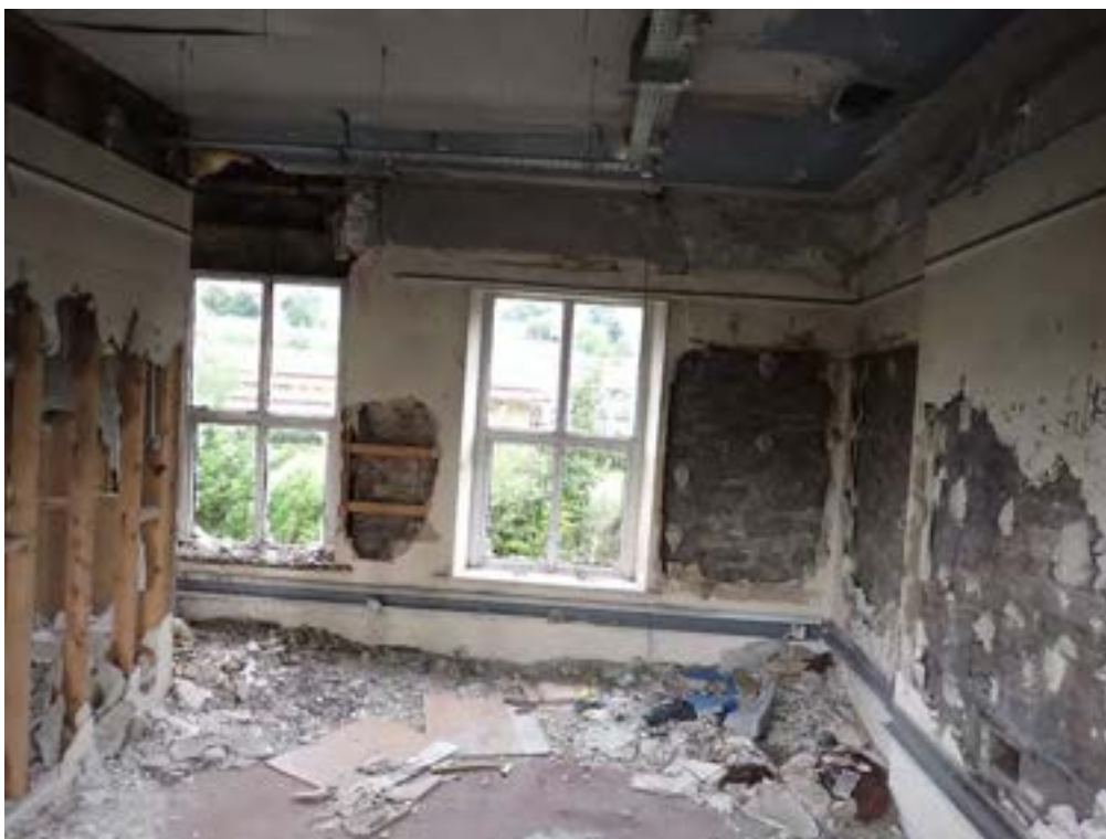
Photograph No : 25 Digital Ref: HOMI_HBR_0108 Direction: W Description: General view of first floor of Building A
