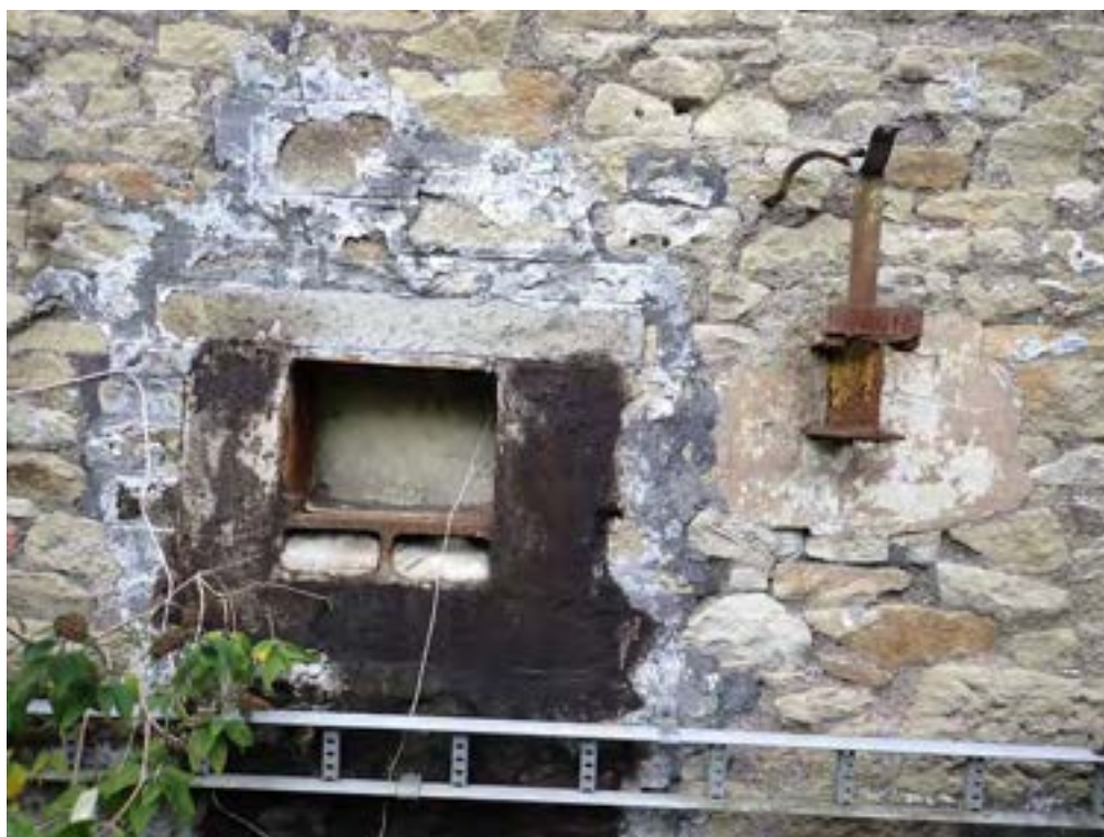
Photograph No : 40 Digital Ref: HOMI_HBR_0103 Direction: N Description: Detail of bearing box and steel I-beam in south gable of Building B
