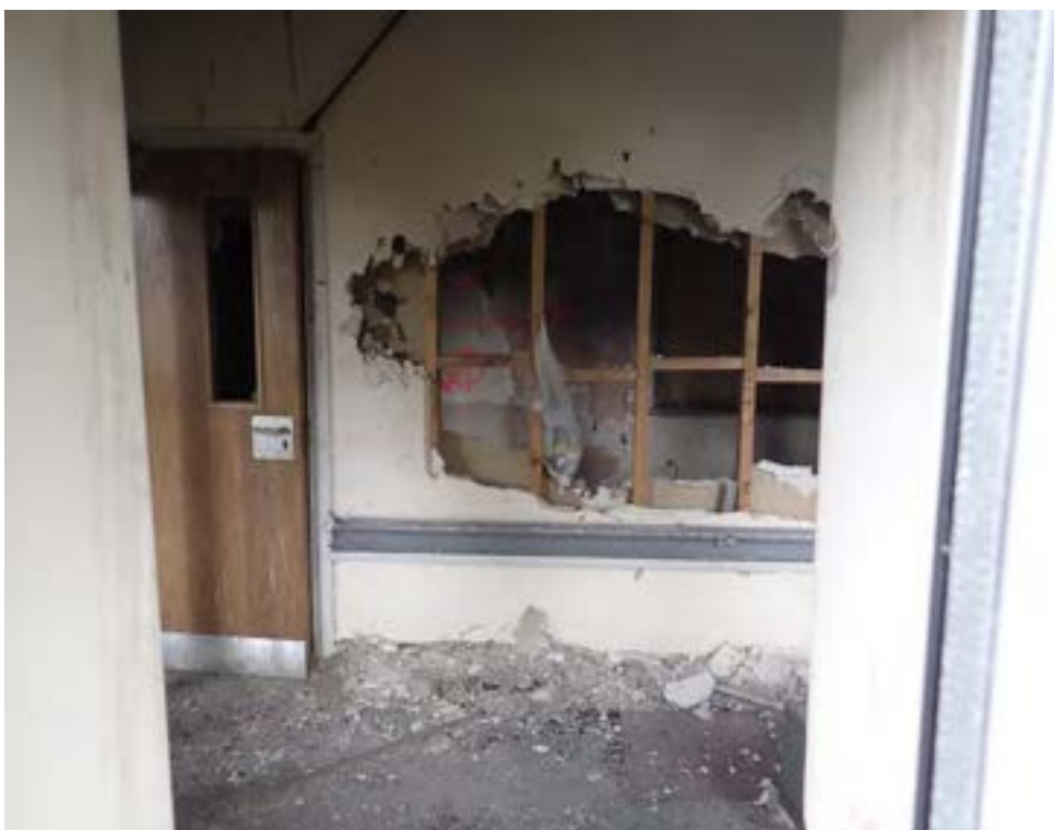
Photograph No : 24 Digital Ref: HOMI_HBR_0105 Direction: W Description: General view of first floor of Building A
