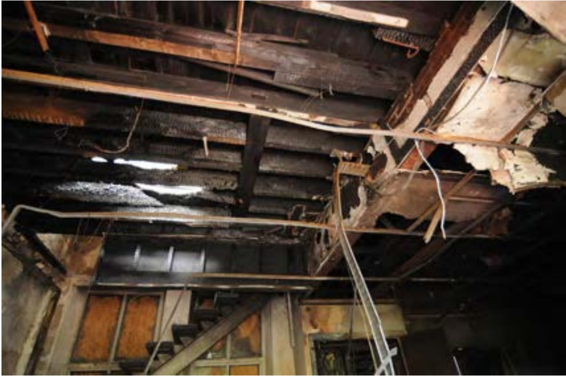
Photograph No : 21 Digital Ref: HOMI_HBR_0069 Direction: W Description: Ground floor ceiling timber beams in Building A
