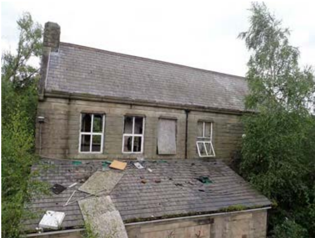
Photograph No : 16 Digital Ref: HOMI_HBR_0110 Direction: SE Description: Chimney, ridge, and first floor windows on west elevation of Building A
