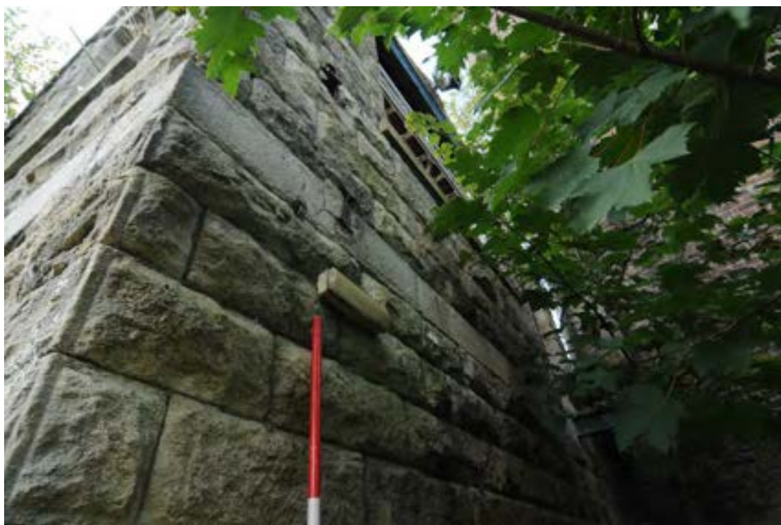
Photograph No : 66 Digital Ref: HOMI_HBR_0020 Direction: SW Description: Detail of ashlar band in north elevation of Building C with large window on first floor
