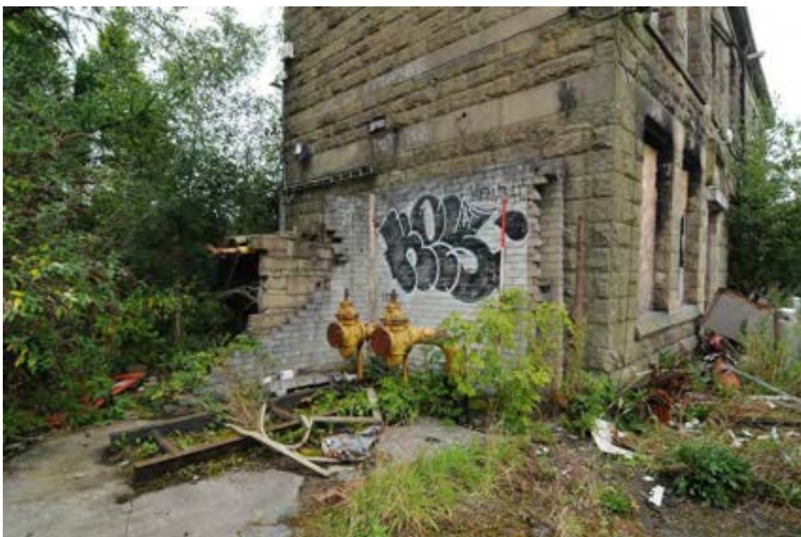
Photograph No : 18 Digital Ref: HOMI_HBR_0086 Direction: SW Description: Brick and stone addition at south gable of Building A with gas
