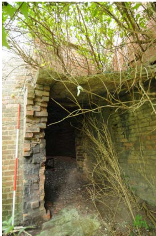
Photograph No : 88 Digital Ref: HOMI_HBR_0028 Direction: NE Description: Opening in south side of chimney and west elevation of Building C (right)
