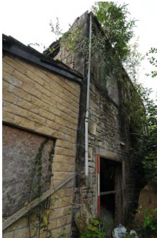
Photograph No : 28 Digital Ref: HOMI_HBR_0057 Direction: SW Description: Quoins at NE corner of Building B with extension in foreground
