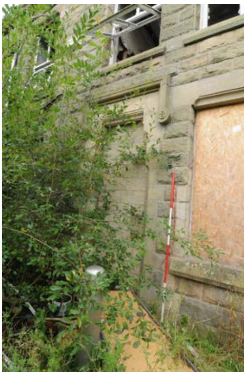
Photograph No : 13 Digital Ref: HOMI_HBR_0076 Direction: SW Description: Stone blocked doorway in east elevation of Building A
