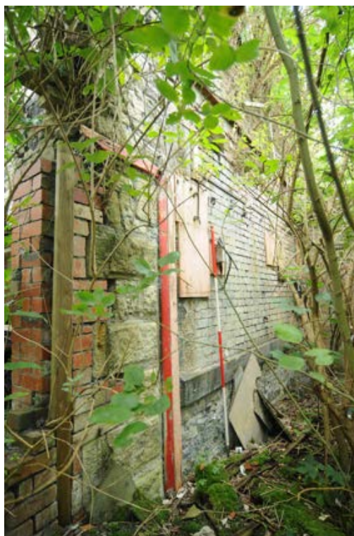
Photograph No : 31 Digital Ref: HOMI_HBR_0116 Direction: NW Description: Southern extent of east elevation of Building B with quoins at extent
