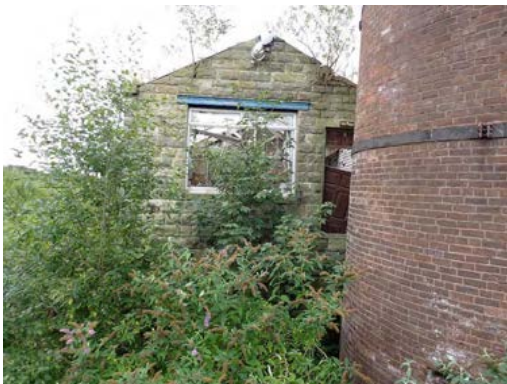
Photograph No : 68 Digital Ref: HOMI_HBR_0096 Direction: S Description: North gable of Building C with Chimney at NW (right)
