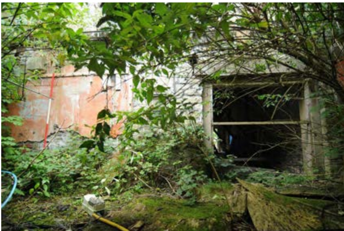
Photograph No : 37 Digital Ref: HOMI_HBR_0127 Direction: N Description: Fenestration in ground floor of south gable of Building B
