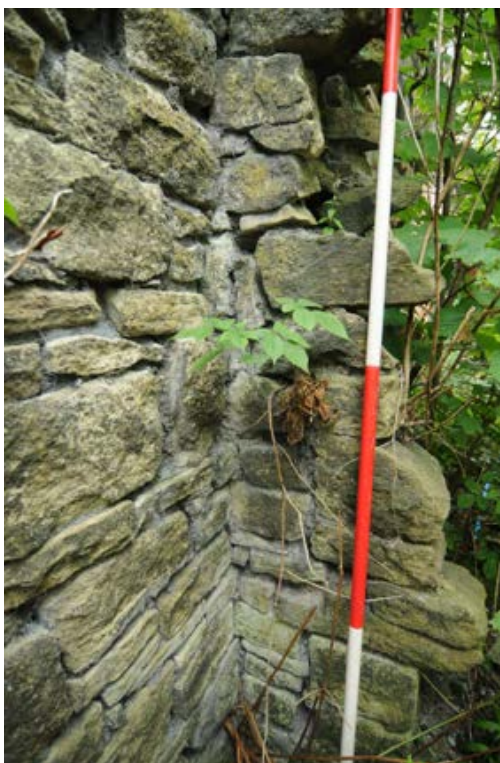
Photograph No : 35 Digital Ref: HOMI_HBR_0131 Direction: NE Description: Detail of south projecting stone wall in south gable of Building B
