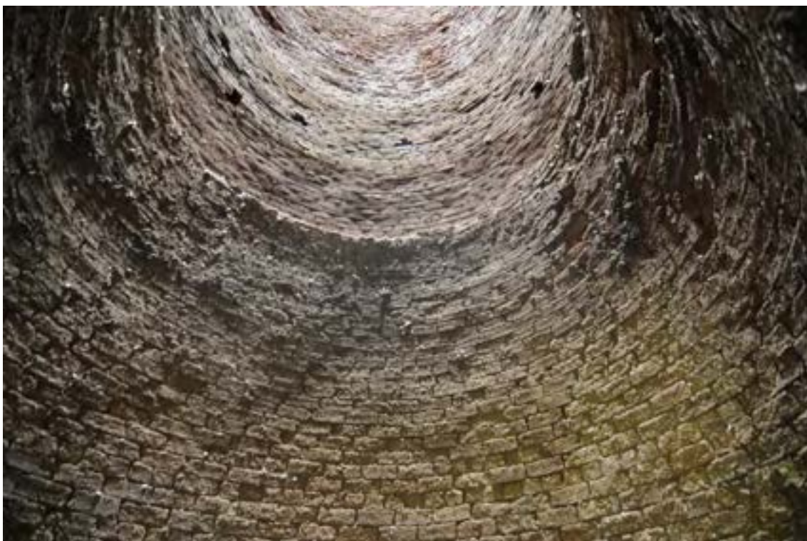
Photograph No : 93 Digital Ref: HOMI_HBR_0033 Direction: N Description: Ledge in internal chimney
