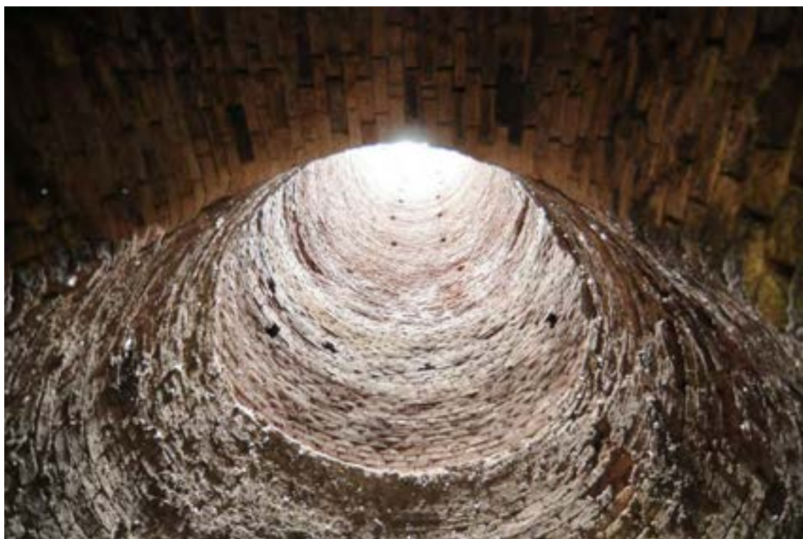
Photograph No : 92 Digital Ref: HOMI_HBR_0032 Direction: N Description: Internal view of chimney
