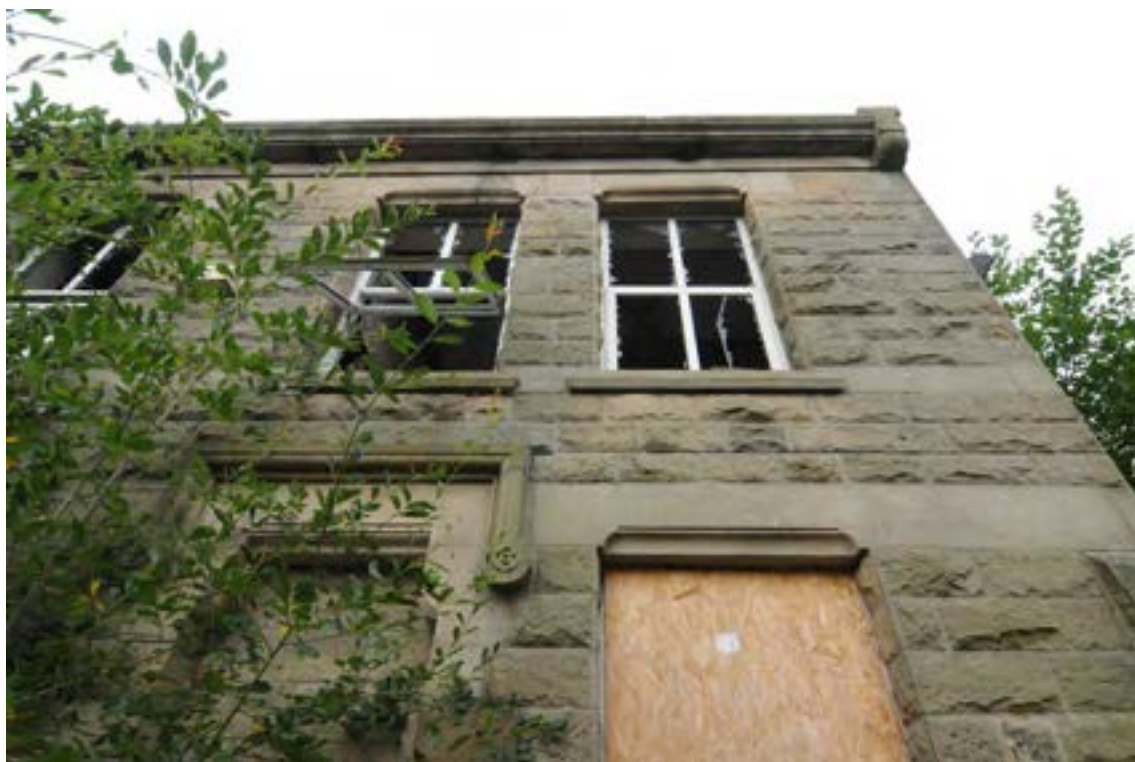
Photograph No : 12 Digital Ref: HOMI_HBR_0077 Direction: W Description: First floor of east elevation of Building A
