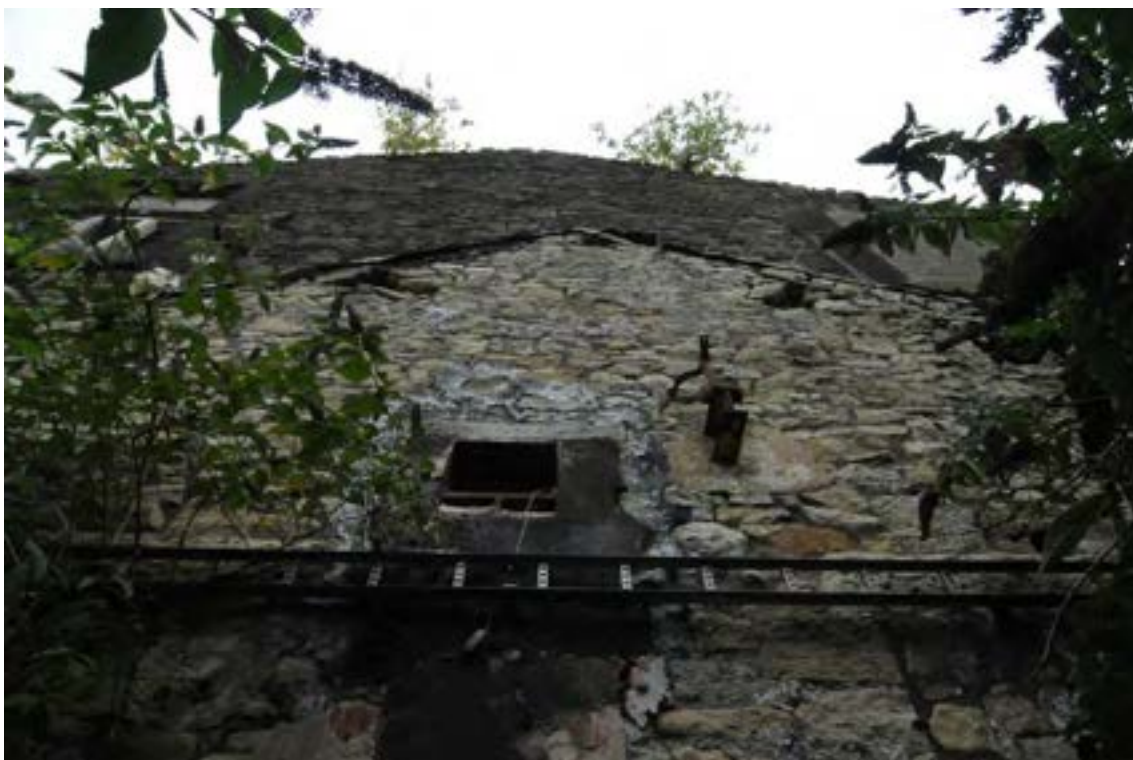
Photograph No : 39 Digital Ref: HOMI_HBR_0119 Direction: N Description: South gable of Building B with bearing box, steel I-beam, gable scar
