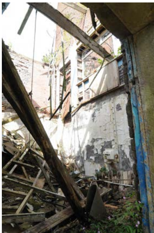
Photograph No : 81 Digital Ref: HOMI_HBR_0016 Direction: NW Description: NW view into ground and first floor of Building C
