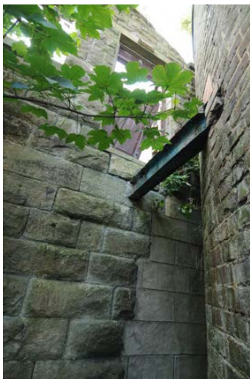
Photograph No : 72 Digital Ref: HOMI_HBR_0021 Direction: SW Description: Door at first floor and blocked opening at ground floor in north elevation of Building C with Chimney to north (right)
