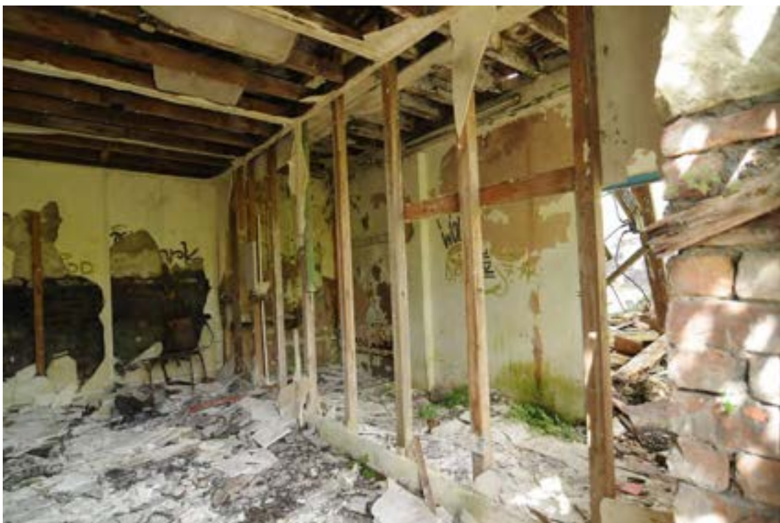
Photograph No : 77 Digital Ref: HOMI_HBR_0011 Direction: NW Description: NW view into ground floor of Building C
