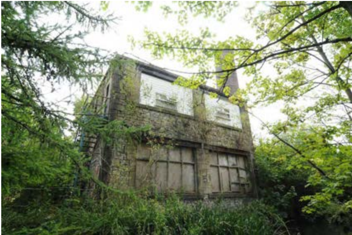
Photograph No : 27 Digital Ref: HOMI_HBR_0061 Direction: SE Description: West elevation of Building B with Chimney in background
