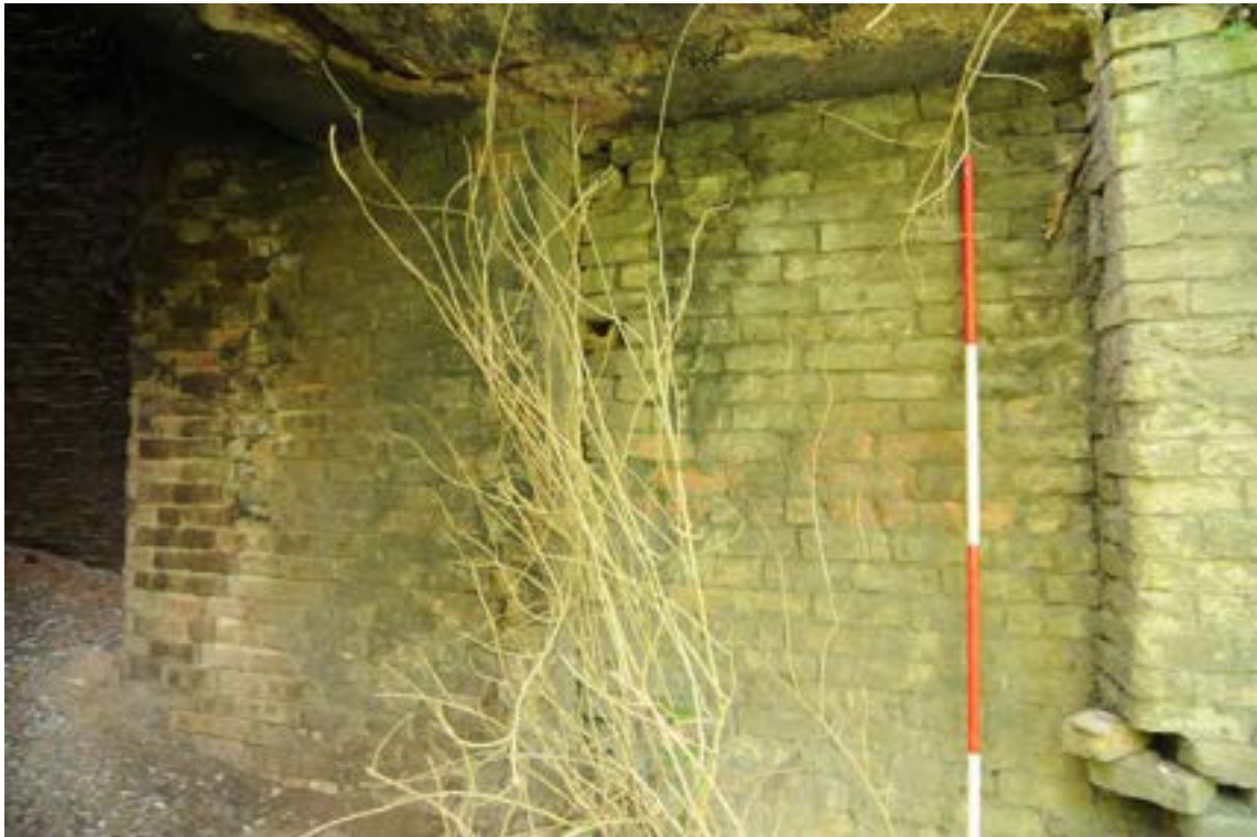
Photograph No : 89 Digital Ref: HOMI_HBR_0029 Direction: NE Description: Opening in south side of chimney and west elevation of Building C (right)
