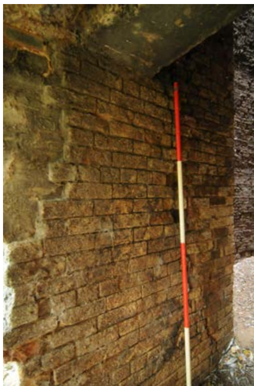
Photograph No : 91 Digital Ref: HOMI_HBR_0031 Direction: NW Description: West wall in opening in south side of chimney
