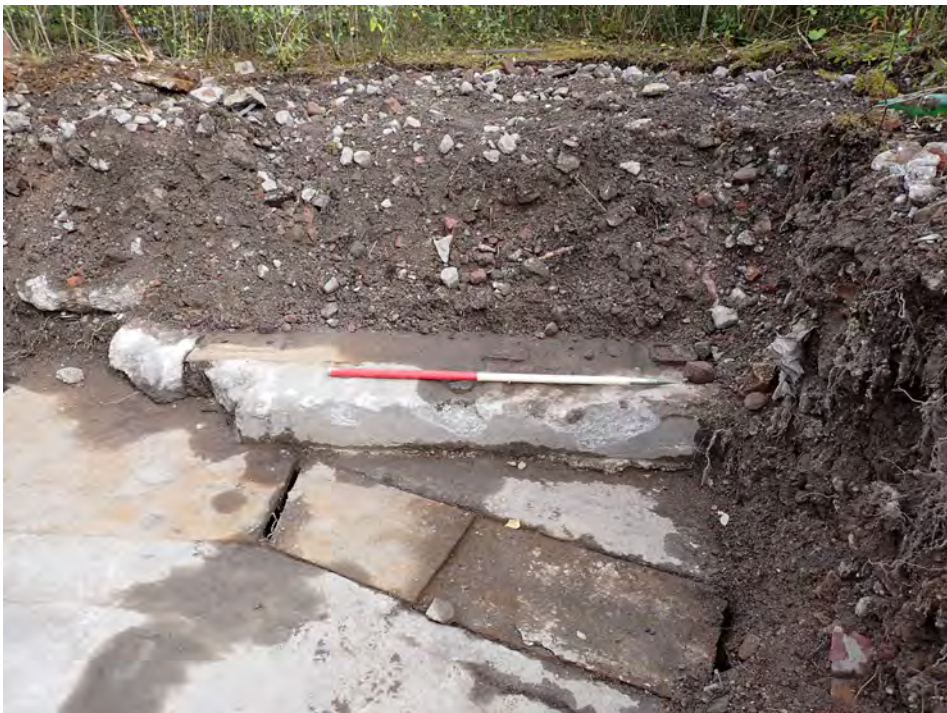
Fig. 4.8: Concrete Floor 202 and Culvert 203
