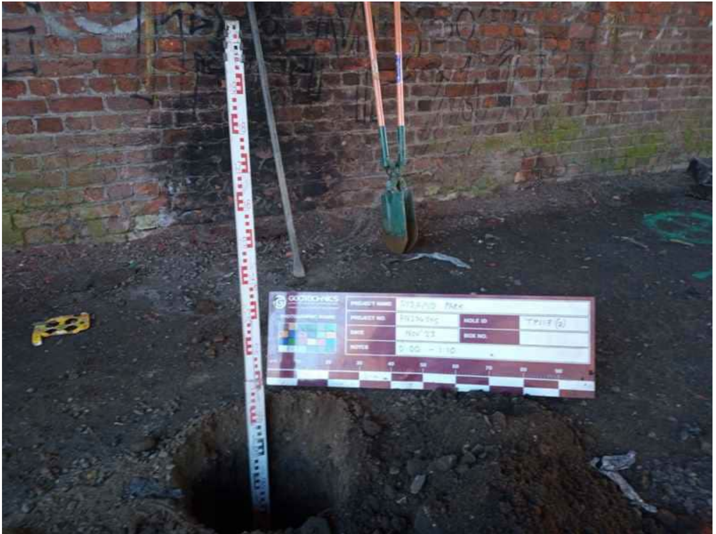
Trial Pit HPI17W (1)
