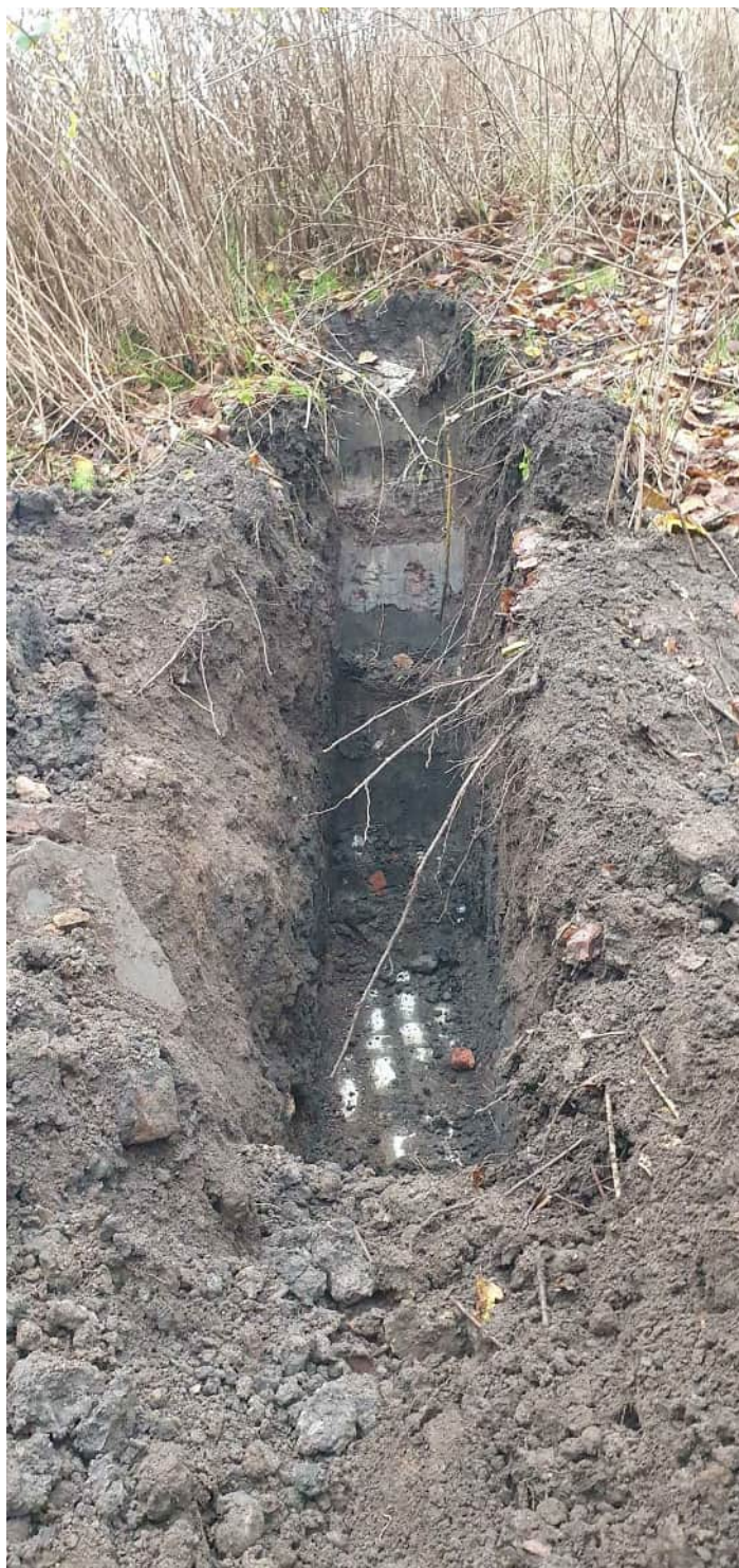
Trial Pit TPI 19 (I)
