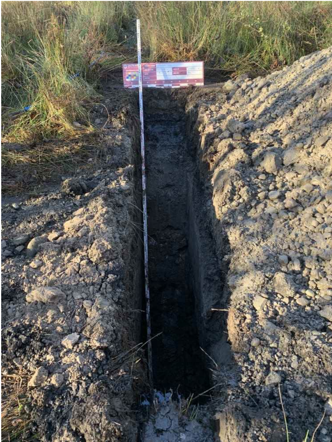
Trial Pit TPI23 (I)
