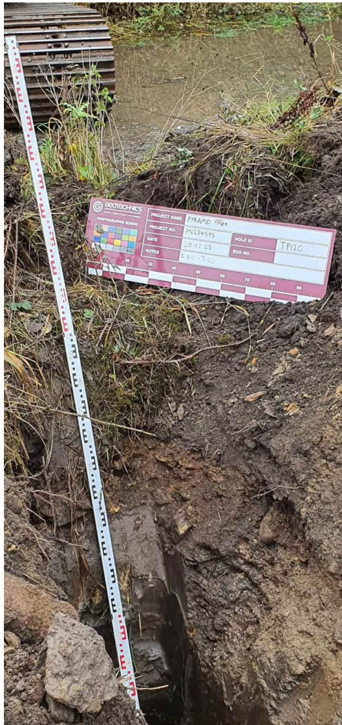
Trial Pit TPI20 (I)
