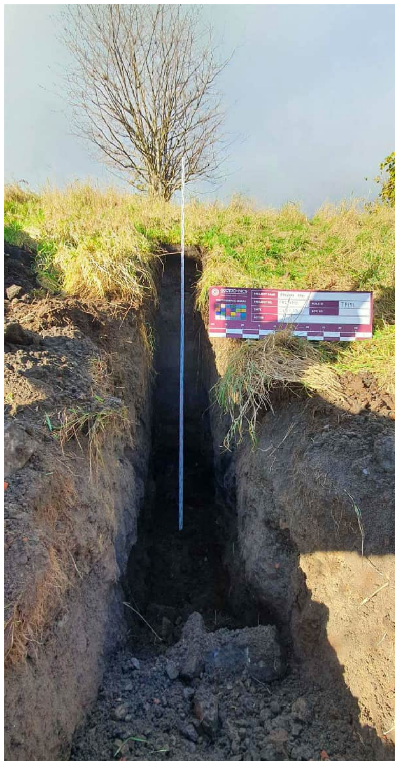
Trial Pit TPI02 (I)
