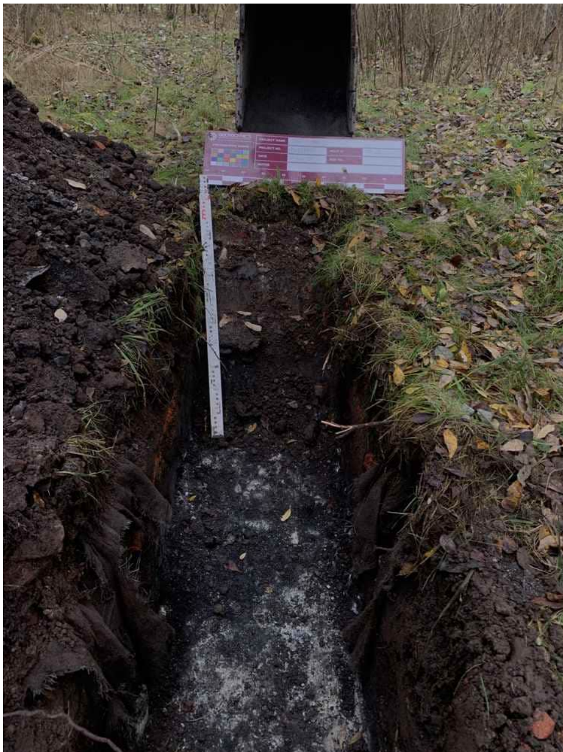
Trial Pit TPI22 (I)
