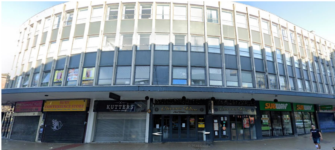
Image 2 – Side view of Lester House from Broad Steet
