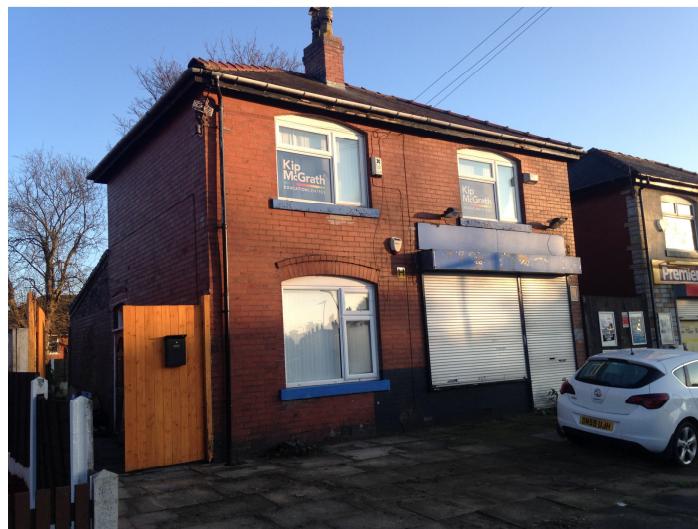
Front elevation with roller shutters indicating the shop part
