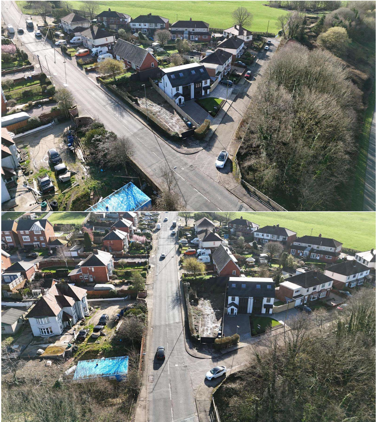
Site in the street from Bury New Road.
