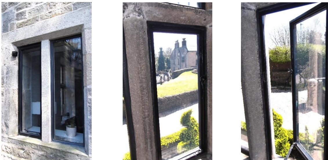
Touchstone windows at Higher House, Holcombe
