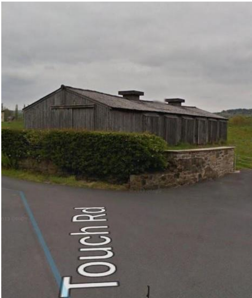
Figure 7 | Existing chicken shed prior to collapse
