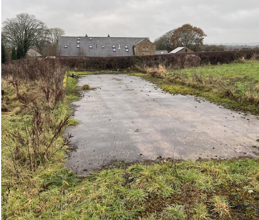
Figure 6 | Existing slab serving former chicken shed
