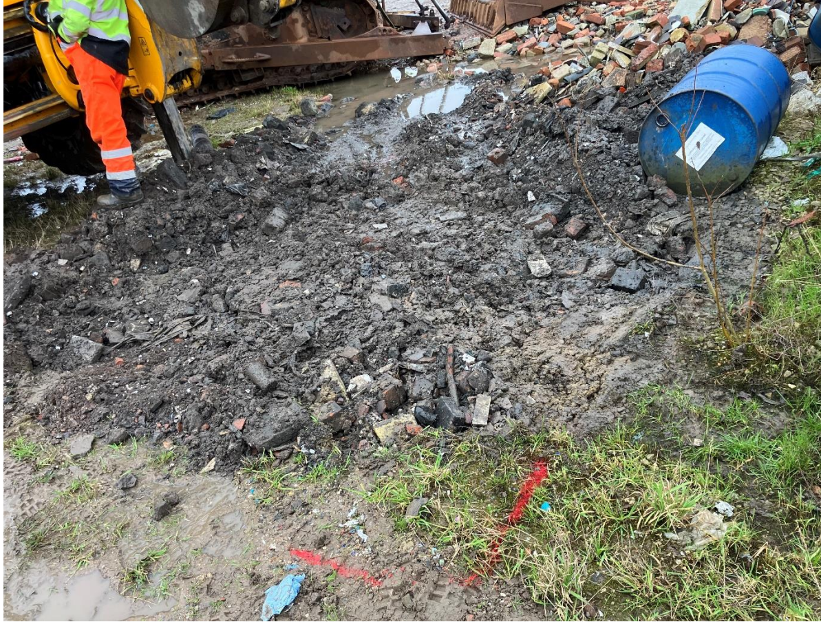
TP08 – Backfilled pit
