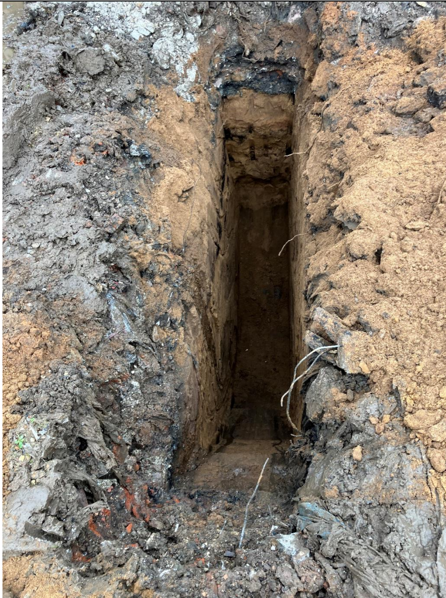
TP02 – Finished trial pit
