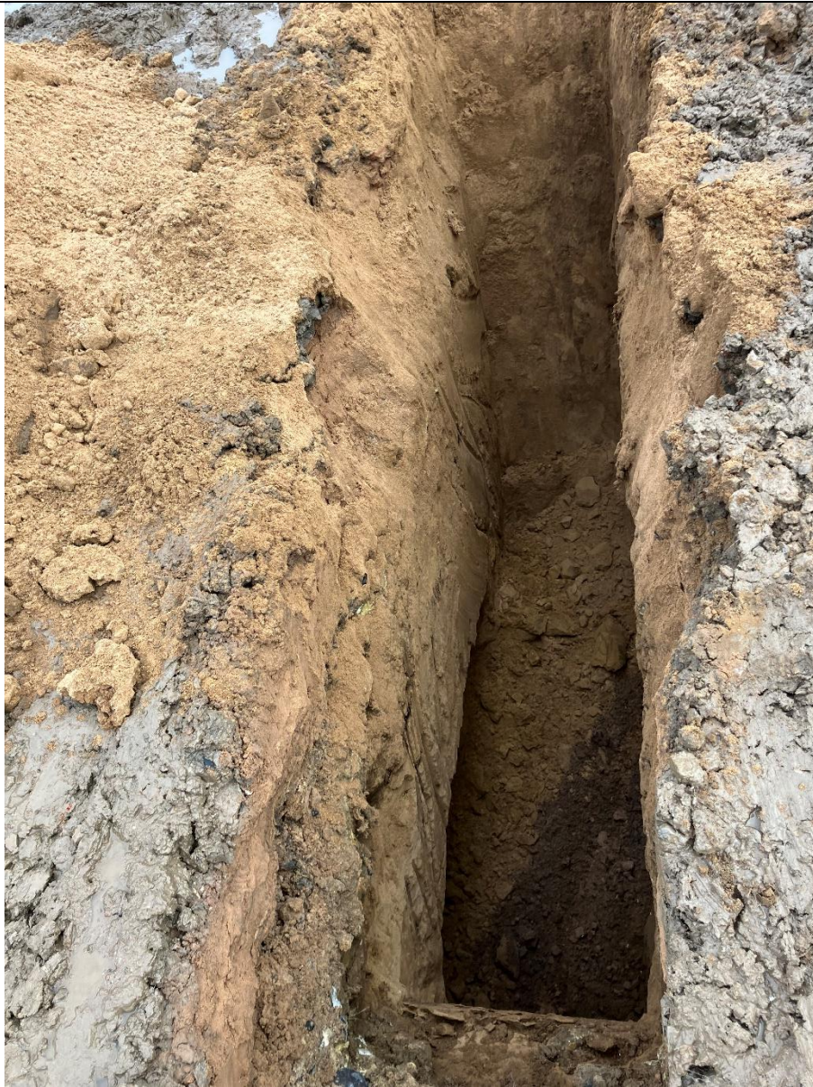
TP06 – Finished trial pit
