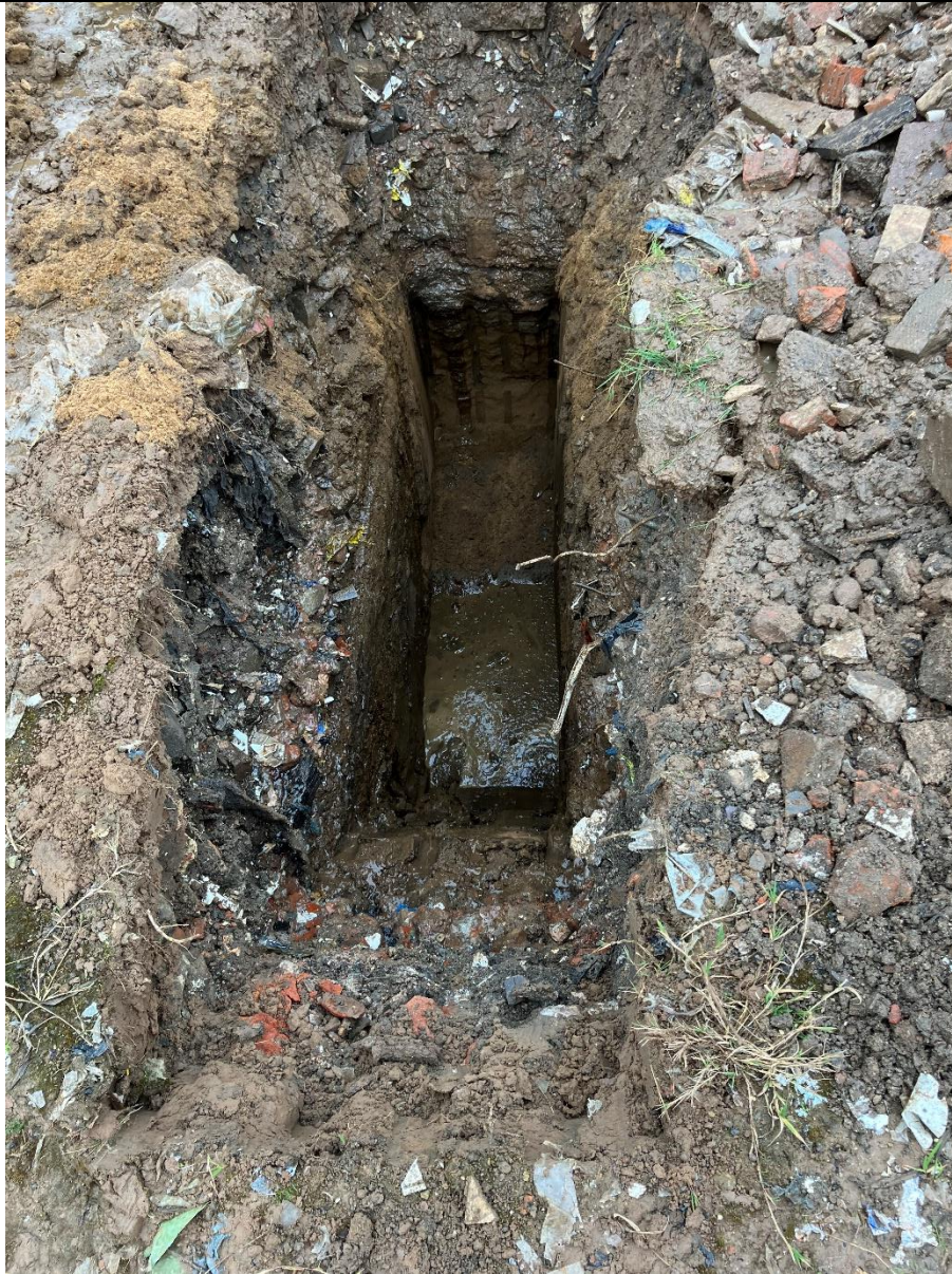
TP03 - Finished trial pit
