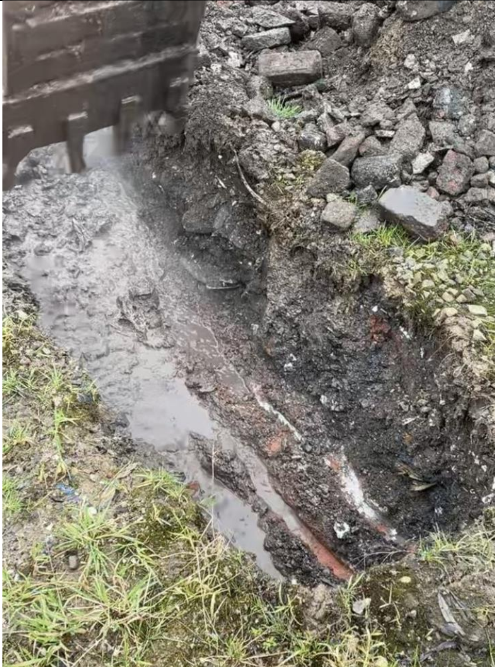
TP08 - Finished trial pit
