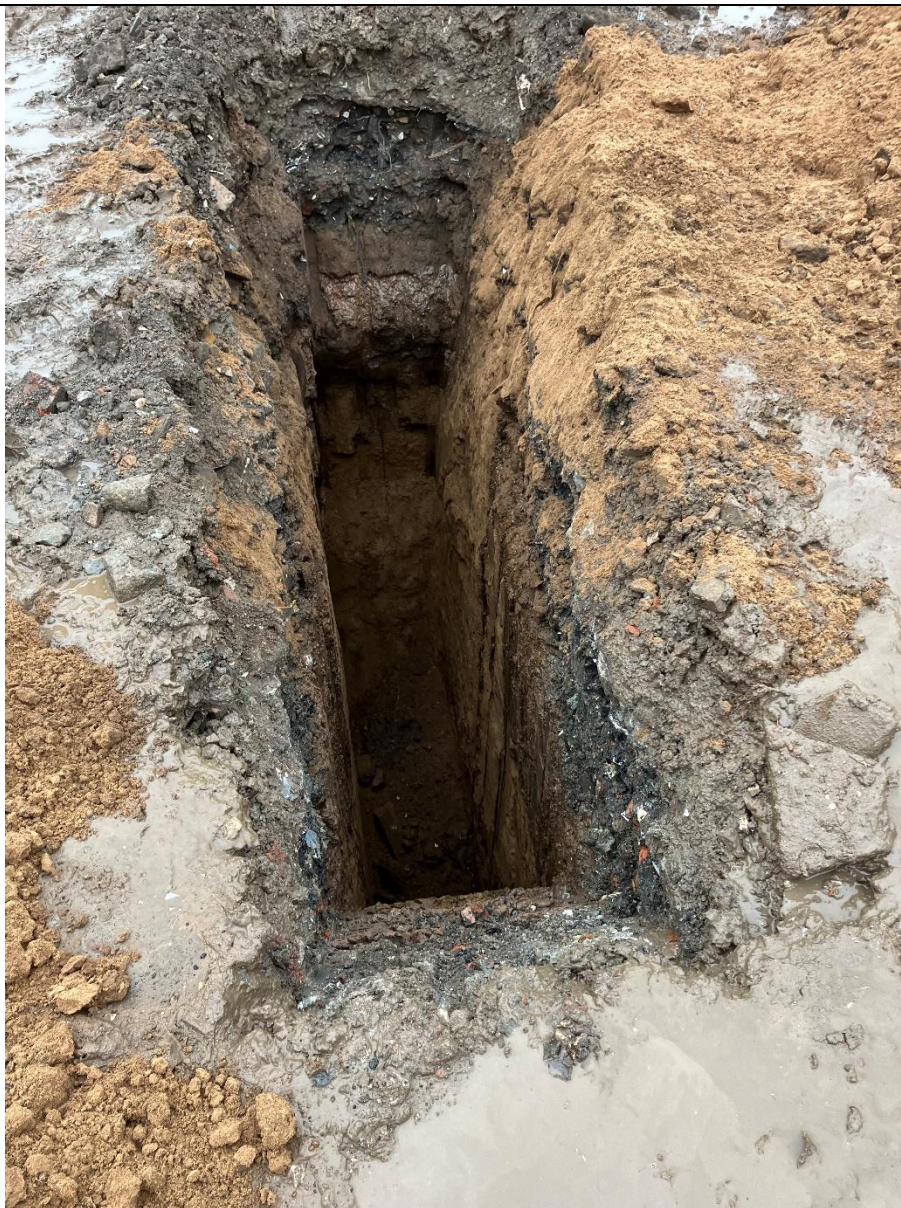
TP01 – Finished Trial Pit
