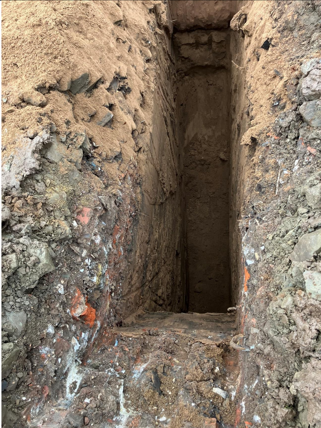
TP04 – Finished trial pit
