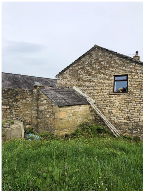
Photograph 1: Overview of the south elevation and the outbuilding where the two story extension is proposed.
