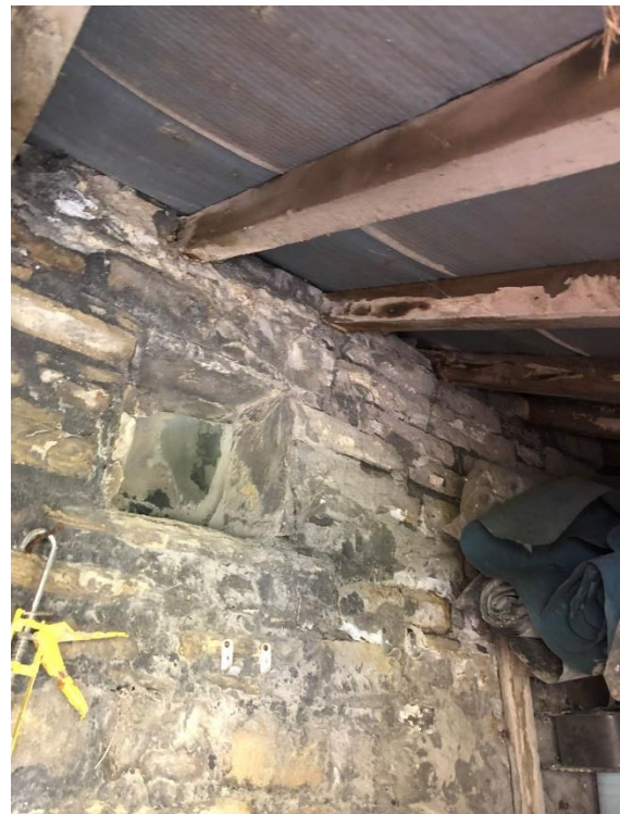
Photograph 8: View inside the outbuilding with wooden truss and roof underlay.
