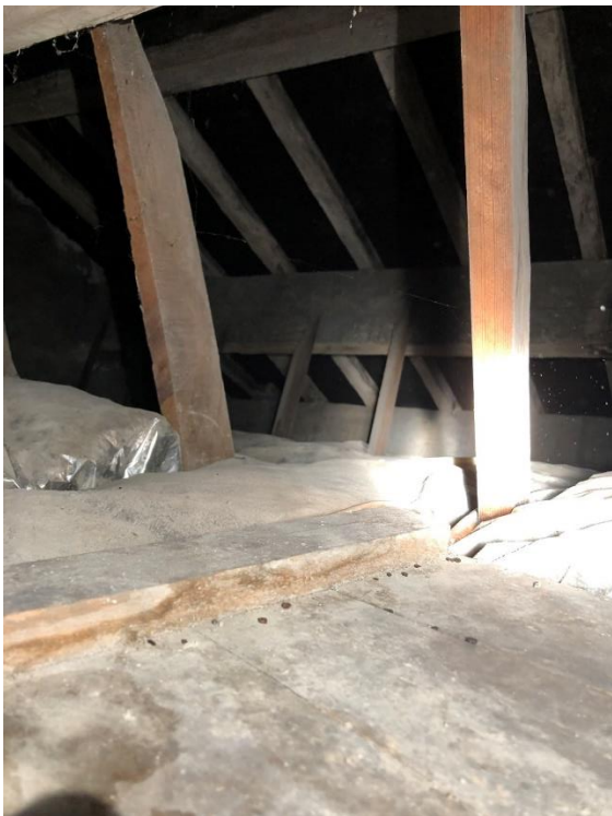
Photograph 6: View of the loft space which had mouse droppings. No bat evidence recorded.
