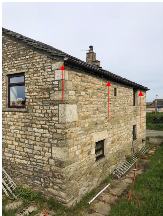
Photograph 2: View of the east elevation with gap present between stone wall and fascia.
