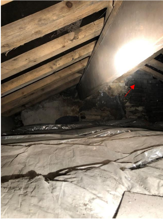
Photograph 5: Wooden roof truss supporting the stone flags. Internal brick wall observed.
