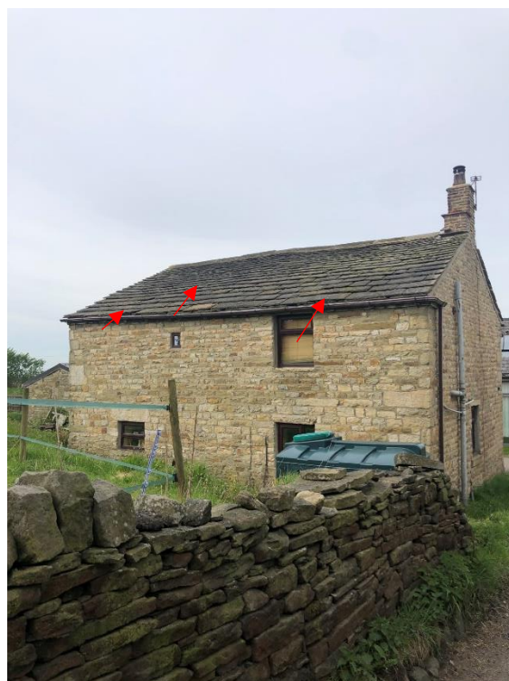
Photograph 4: View of the east elevation. Stone roof has gaps between flags.
