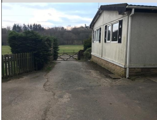
Photograph 7: Bungalow located in the west and a gate to fields in the south.
